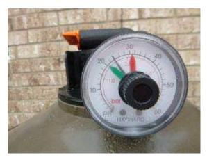
The pool filter was a <u>cartridge</u> filter that was functional at the time of the inspection, and showed an operating pressure of 22 psi. This is within a normal range of operation, and no repairs are recommended.
