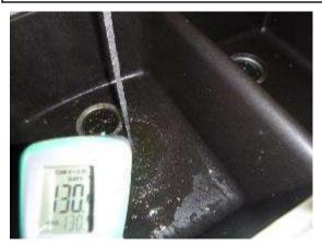
The water temperature was checked at the kitchen sink. The water temperature was observed to be hotter (130F) than recommended (120F) and this is considered a scald risk. The risk of serious injury is higher when the water heater thermostat is set above 120F. It is recommended that the water heater thermostat be adjusted to prevent safety hazards. (Information)
