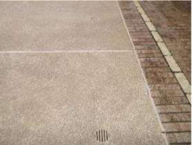
The grading of the yard appeared sufficient to channel rain water away from the pool.
