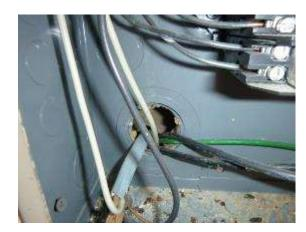
The holes in the panel where the individual circuit enter the panel did not have a bushing or clamp to protect the conductors from the sharp edges of the knock out hole provided and needs repair.
