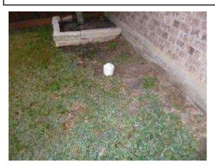
The main sewer PVC clean out was located at the south side of the house. The clean out is needed in the event of a stoppage in the main sewer drain line, and the clean out is where a sewer snake would be installed to remove the clog in the drain line.
