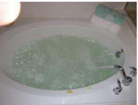
The whirlpool tub was functional at the time of the inspection, however the on/off push button for the whirlpool tub sticks and needs to be repaired.
