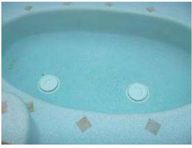
The bottom drains for th spa contained two inlets, which reduces the potential hazard for entrapment.
