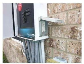
The pool and spa lights were functional at the time of the inspection, and were protected by a Ground Fault Circuit Interrupt device, which was also functional at the time of the inspection. (Information)
