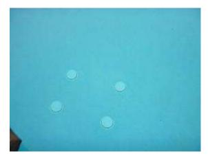
The bottom drains for the pool contained four inlets, which reduces the potential hazard for entrapment.
