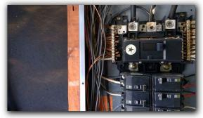
Mhite "neutral" type wiring used as "hot" needs to be properly identified as "hot" in panel box at one or more locations. White wiring should be wrapped with black tape or marked with a black (or other appropriate color that is not white, grey or green) marker.
