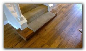
☑ Improper dimensions of stair risers: riser height cannot vary more than 3/8" from the lowest riser to the top riser per current code. (See IRC 2015, R311.7.5.2)
