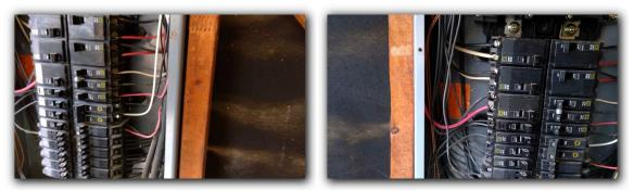
White "neutral" type wiring is required by current code to be individually secured into individual holes in "neutral" buss bar. Double wiring and securing two or more wires to a single set screw is not allowed per current code on the "neutral buss bar.
