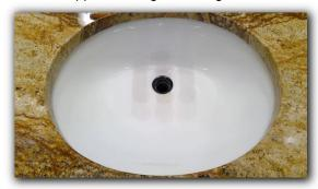
☑ Sink stopper missing or damaged in master bath sink left side
