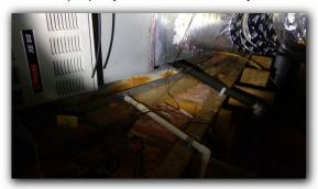
☑ Metal shroud on the right side of the house behind the HVAC condensing units is not properly installed on the exterior wall.
