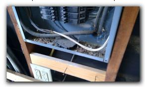
☑ Panel box does not conform to current code regarding the proper presence of arc fault protection. Arc fault protection did not enter the NEC code until 2002.
