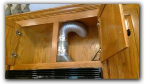
A Range hood vent exhaust termination point present that appears to be an old range hood vent piping termination point from a pre-remodel location. The new one is located on the perpendicular wall around the corner from the old one.
