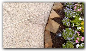
☑ Cracks observed in the mortar / grout joints / tile of the swimming pool tile. Cracks should be filled to prevent erosion between the swimming pool deck and coping.
