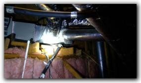
☑ Master closet is a "walk in" type closet but is not serviced (ducted) with a supply register. While this is not a "design" inspection. It is a usual and customary building practice to supply air conditioning and heating to these spaces.
