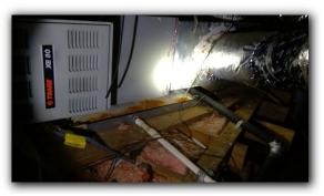
☑ Secondary drain pan for the smaller HVAC evaporator coil in the attic space is not properly located. The pan should extend a minimum of 2" past the evaporator coil on all sides. Pan should be properly located to catch any condensation from the evaporator coil if needed.
