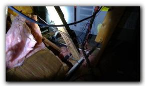
☑ Refrigerant lines not properly insulated at evaporative coil (wrong thickness per current code)
