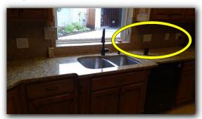
House does not conform to current code regarding proper receptacle placement: Receptacles required servicing countertop space 12" or greater per current code.
