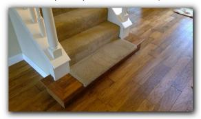
☑ Hand railing is not continuous. Current code states that the handrail can only be interrupted by a newell post at a turn. (See IRC 2015, R311.7.8.2, Exception 1.)
