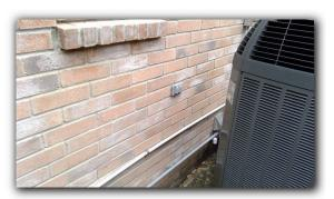
☑ Loose, damaged, missing outlets / switches /covers at one or more locations.
