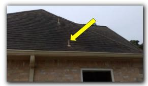
☑ Flashing is lifting, ill configured, or missing
