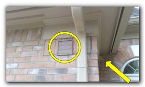
☑ Range hood / exhaust vent appears to be cracked / broken.
