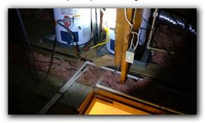
☑ 30" working clearance and platform needed in front of water heating equipment per current code.
