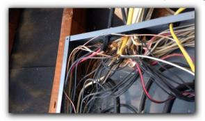
☑ Wiring from the disconnect to the HVAC condensing unit #1 appears to be #10 wiring which is rated for a maximum of 30 amps. Unit max and minimum circuit breaker is 60 amps.
