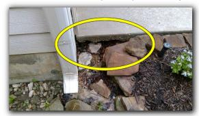
☑ Nuts and washers need to be installed on j-bolts connecting the sill plate to the concrete foundation (multiple locations). (IRC 2015, R403.1.6)
