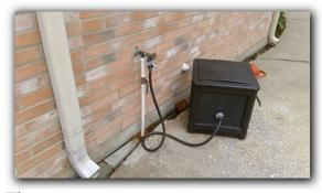
☑ Proper insulation needed on exterior exposed water lines / plumbing
