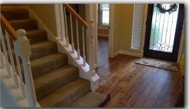
☑ Hand railing does not properly terminate by turning into the wall at handrail ends per current code. (See IRC 2015, R311.7.8.2)
