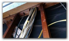
☑ Improper use of extension cords as permanent wiring observed in one or more locations. Permanent use of extension cords for permanent wiring is considered a safety hazard by current standards.
