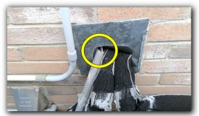
$\square$  Dryer vent is installed too close to exterior HVAC condensing unit. Lint from tthe dryer unit can potentially block the ventilation fins of the condensing unit.
