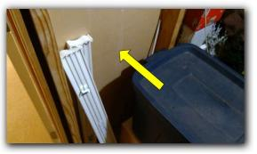
☑ Both air haucs and ridge venting is being used at the same time to ventilate the attic space in some locations. No soffit ventilation is present at the garage and breezeway areas. The use of air haucs and ridge venting at the same time is not an effective ventilation system as air can be drawn from the air haucs into the ridge vents without proper cross ventilation in the attic spaces.
