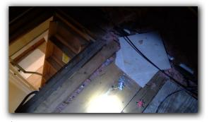
☑ Voids observed in insulation in attic space at one or more locations.
