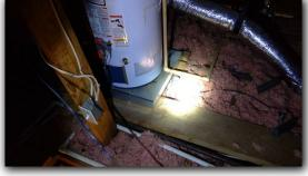
☑ Sediment trap not present in gas line at water heating equipment
