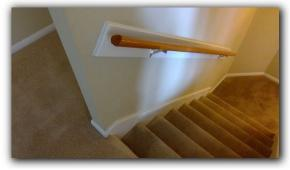
☑ Hand railing not at proper height: Current code requires handrail to be installed 34" to 38" measured vertically from the bullnose of the stairs. (See IRC 2015, R311.7.8.1)
