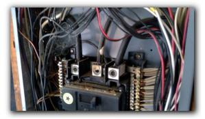
☑ Panel covers, knockouts, cable clamps missing/ loose in panel box at one or more locations.
