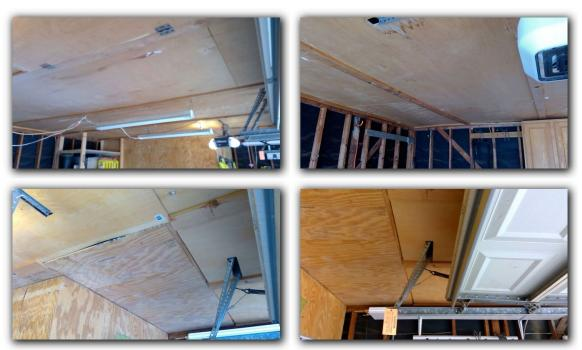
☑ Proper 30" working clearance and level platforms needed in front of equipment located in attic space at one or more locations.
