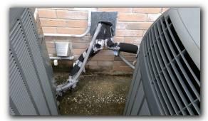
☑ Conduit is not properly connected / installed at exterior brick wall
