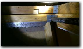
Proper fire separation needed between garage and attic space. Wood present in the ceiling of the garage is not appropriately fire rated.
