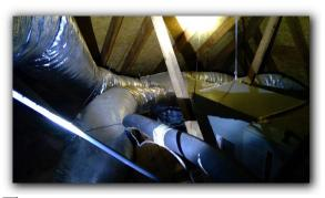
☑ Refrigerant line insulation at condenser unit(s) is deteriorated
