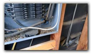
Ground and neutral wiring intermingled on the same buss bar in panel box at one or more locations.
