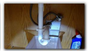
☑ Evidence of previous water leaks present under bathroom sink locations.
