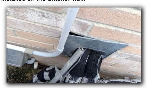
Refrigerant lines not properly insulated at evaporative coil. First 12 feet of the primary drain line should be insulated.
