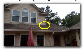
${\ensuremath{\,\overline{\square}}}$  Flashing / counterflashing not properly caulked
