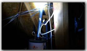
☑ Electrical Romex type wiring has not been properly stapled above panel boxes and junction boxes at some observable locations
