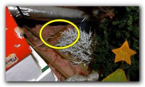
☑ Voids observed in insulation at knee walls in attic space at one or more locations.
