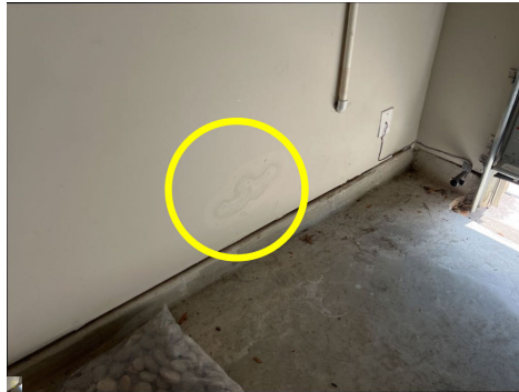
Water stain on the north interior garage wall.
