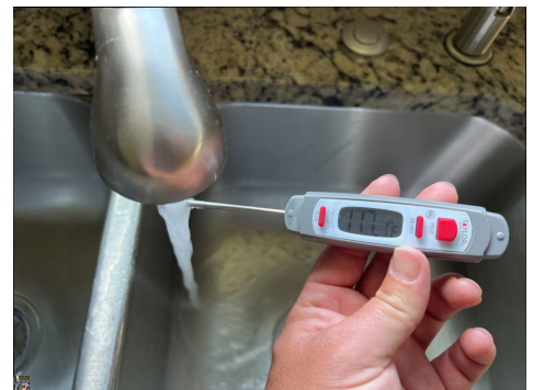
Hot water temperature test during the gas reinspection.
