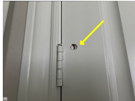
Door damaged at the master water closet
