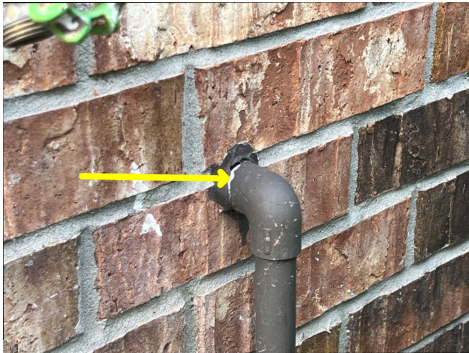
Seal all exterior penetrations.
