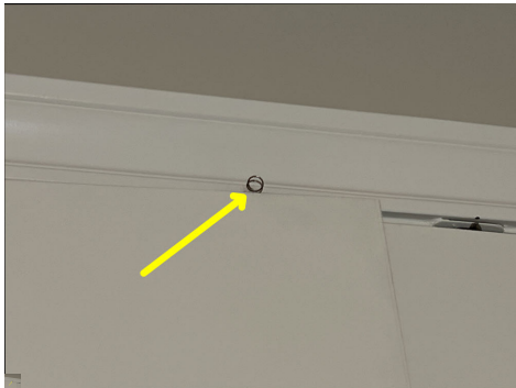
Ball latch damaged at the top of one or more doors.
