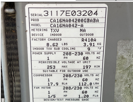
Condenser unit: Carrier 3.5-ton 2017 R-410A
