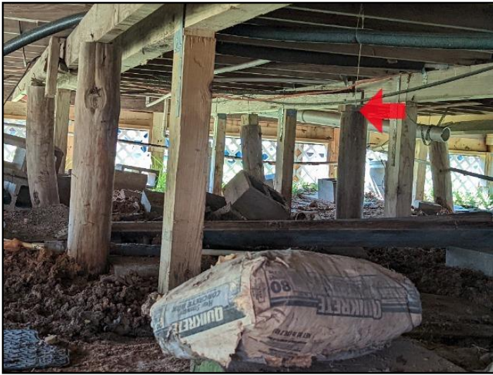
22. Poorly secured at top or bottom
