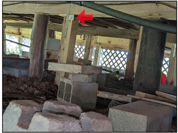
23. Poorly secured at top or bottom
