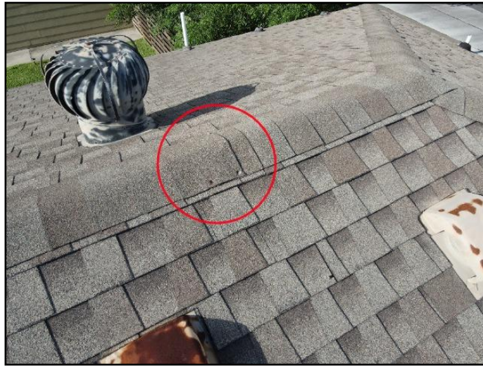
6. Exposed fasteners
