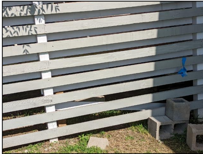
20. Boards damaged
