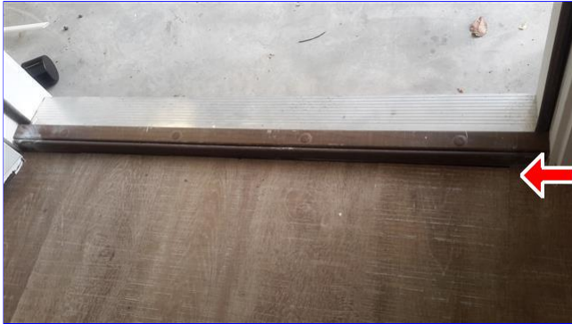
F. Item 3(Picture) 1st floor at garage
