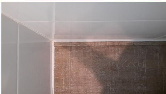
F. Item 5(Picture) master bath behind tub
