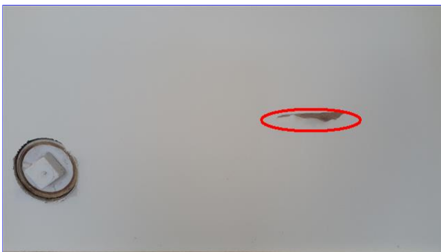
E. Item 27(Picture) garage rear wall
