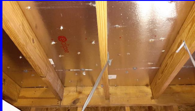
2x6 rafters stick built with radiant barrier decking
