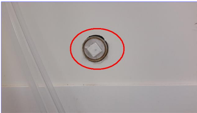
E. Item 11(Picture) garage rear wall
