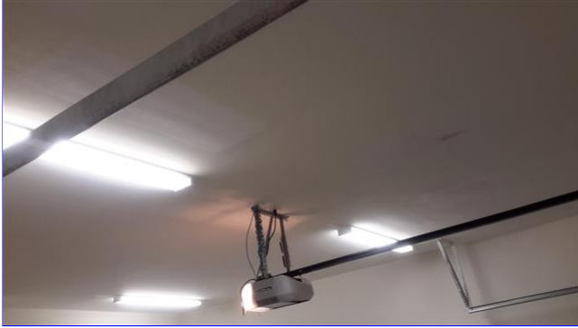
F. Item 2(Picture) garage
