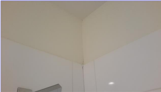
E. Item 17(Picture) 1st floor bathroom
