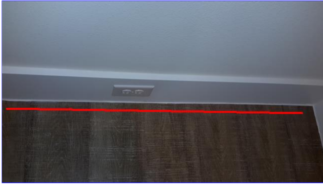
E. Item 5(Picture) 3rd floor rear bedroom
