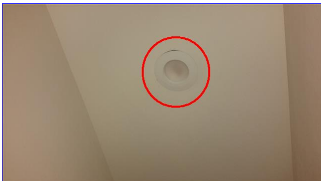
B. Item 3(Picture) 3rd floor rear bedroom closet
