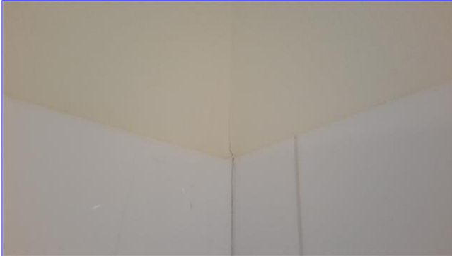
E. Item 18(Picture) 1st floor bathroom
