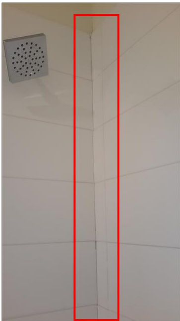
E. Item 28(Picture) 1st floor bathroom
