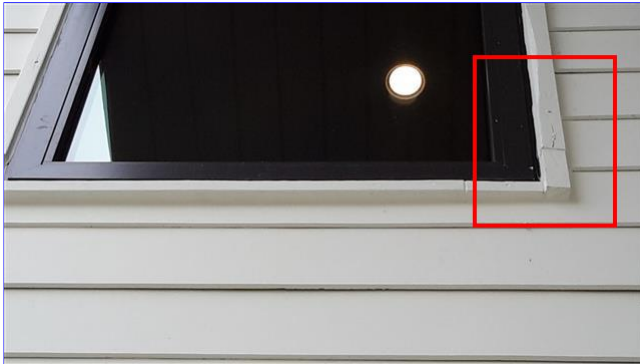
E. Item 8(Picture) 3rd floor right side of home
