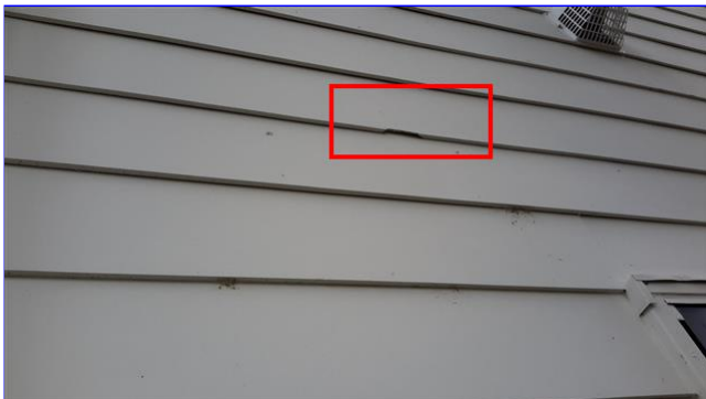
E. Item 9(Picture) Rear of home
