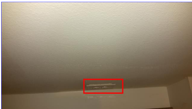
B. Item 1(Picture) Loose outlet stairs to second floor
