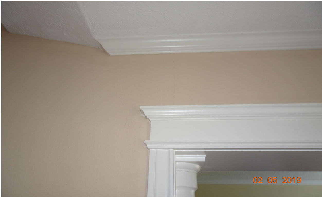
Photo # 16 Crack at ceiling, left side of entry hall diagonal offset corner
