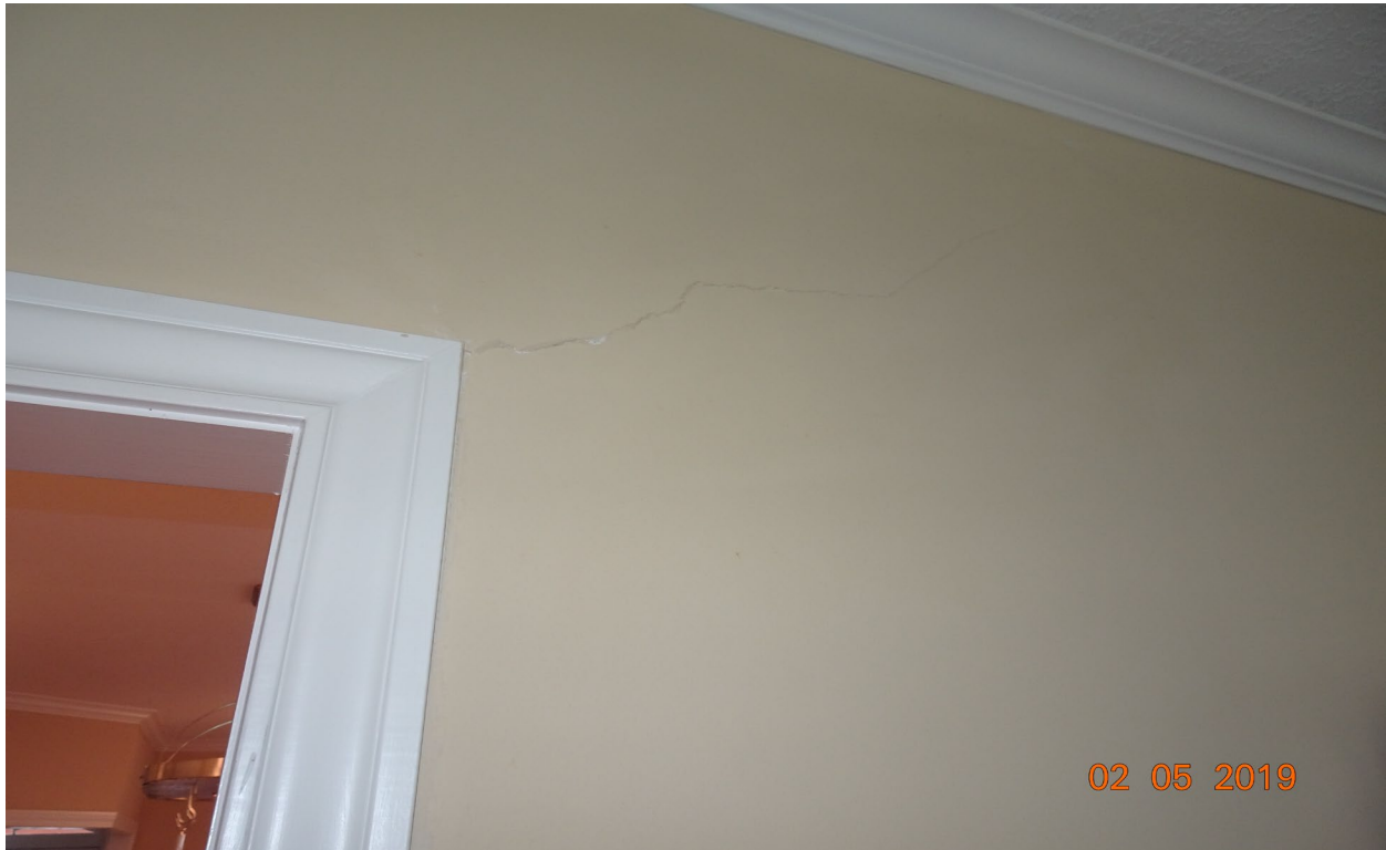
Photo # 20 Crack at top right of door to utility room
