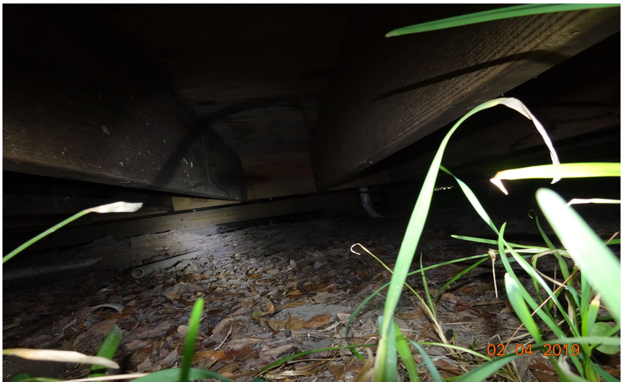
Photo # 6 Crawl space – minimal clearance under beam
