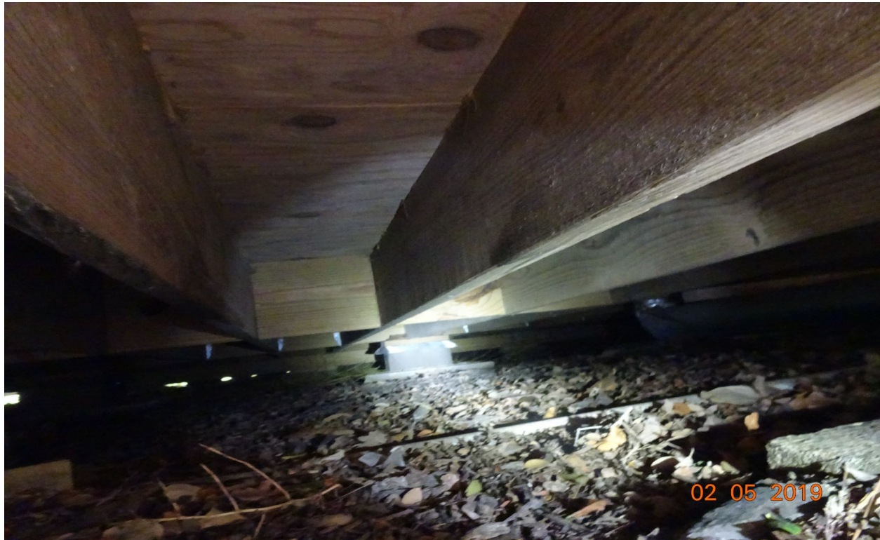
Photo # 14 Crawl space, note wood shims
