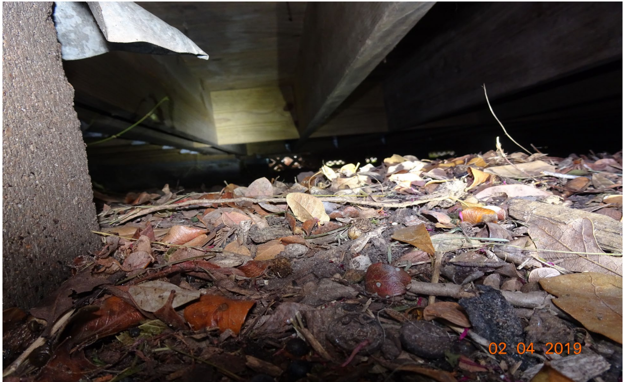
Photo # 6 Crawl space – minimal clearance under beam
