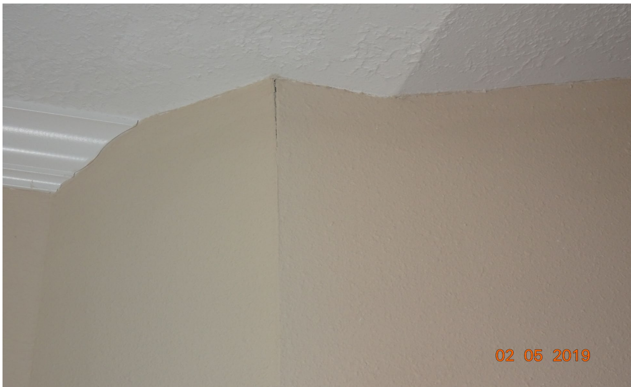
Photo # 16 Crack at ceiling, left side of entry hall diagonal offset corner
