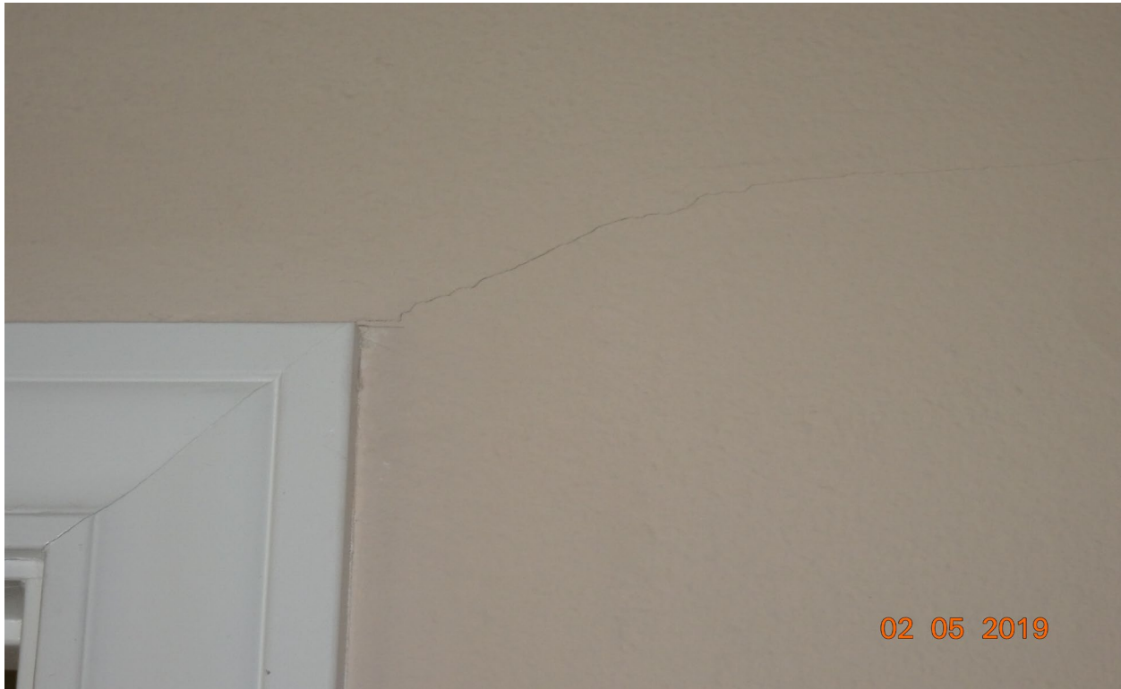
Photo # 18 Crack at left side of “bridge” over foyer
