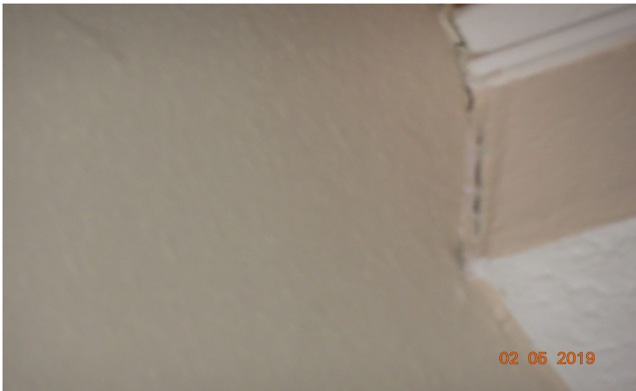
Photo # 18 Crack at left side of “bridge” over foyer
