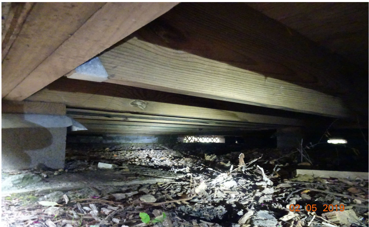
Photo # 14 Crawl space, note wood shims
