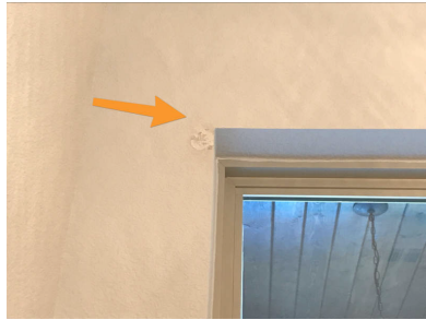
Touch Up At Window Above Front Door
