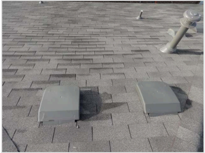
Roof view - side slope
