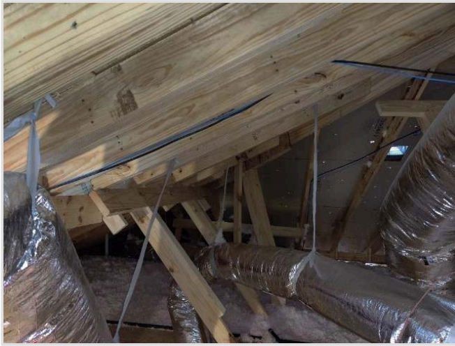
Attic view - framing
