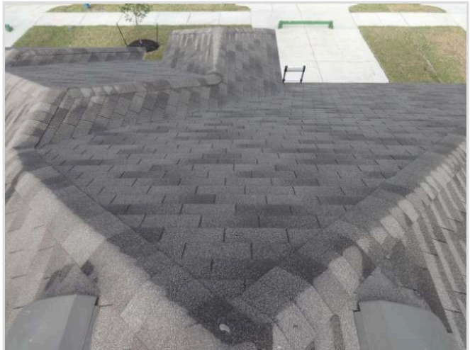
Roof view - front slope
