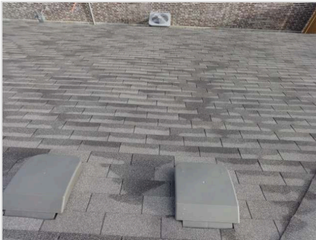
Roof view - side slope
