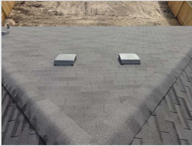
Roof view - rear slope
