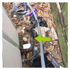
• Exterior condensing unit is out of level, recommend having unit leveled to promote best overall operation and function.
