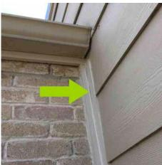
• Exterior walls show typical minor settling cracks, no other visual indications of structural movement were noted at the time of the inspection. Re-point mortar area(s) and seal as necessary to reduce unwanted moisture intrusions and promote good weather seal.
