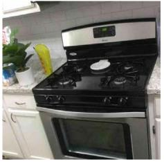
No anti tip device installed on freestanding range. Recommend adding anti-tip device to reduce the possible hazards associated with range tipping. I = Inspected NI = Not Inspected NP = Not Present D = Deficient I NI NP D\* **E. Microwave Ovens** Comments: • Microwave built-in unit functioning as intended at time of inspection. F. Mechanical Exhaust Vents and Bathroom Heaters Comments: • Functioned properly. **G.** Garage Door Operators
