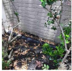
· Vegetation direct contact. Cut back away from siding, roof covering and slab to reduce the amount of moisture close to structure, and to reduce the amount of wear to building materials
