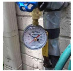
• Galvanized water lines noted in home for the main water supply. These lines can corrode and clog over time reducing or stopping water flow/pressure. While visual evidence at the time of the inspection notes the system is functioning within normal parameters, consider upgrading to PEX pipe to reduce possible failure in lines and related issues.
