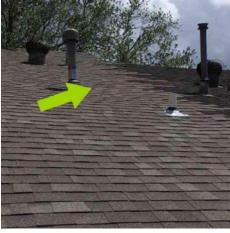
• Missing shingle and granule loss noted. Recommend licensed contractor evaluate and repair or replace.
