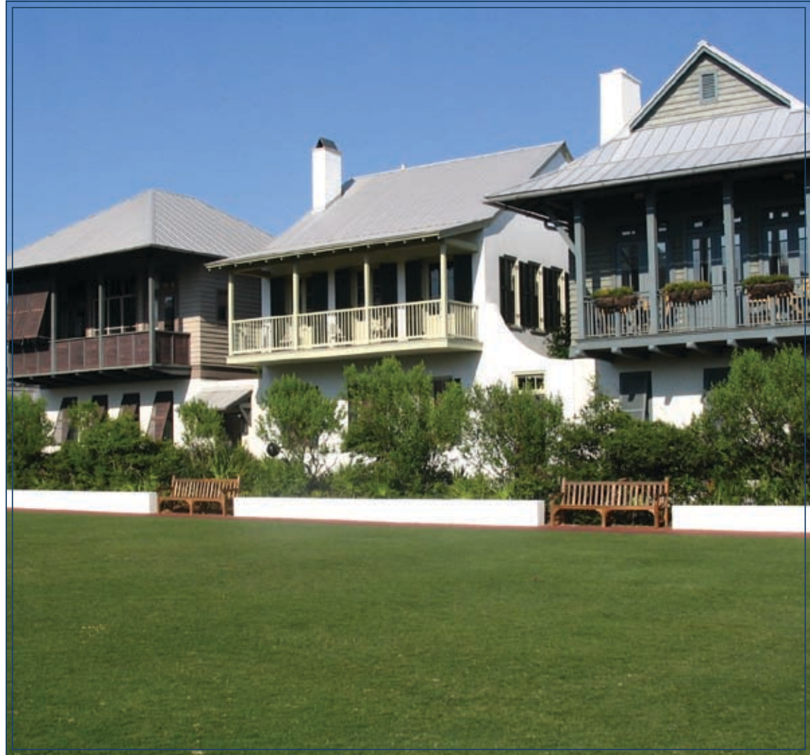
Fig. 4.1: Typical architecture and building proximity.
