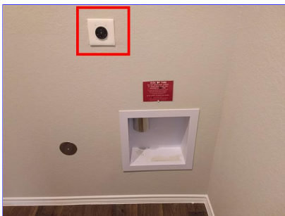
L. Item 1(Picture) laundry room
