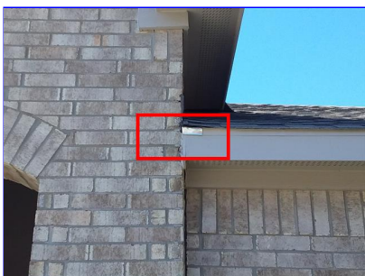
C. Item 3(Picture) front of home
