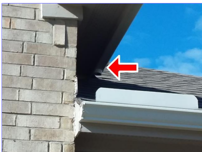
B. Item 2(Picture) roof line areas
