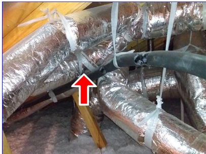
C. Item 1(Picture) multiple areas
