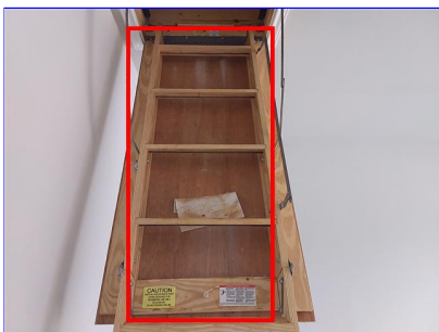
D. Item 1(Picture) garage access
