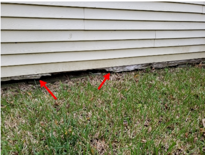
Damaged wood siding underneath vinyl siding on rear of house
