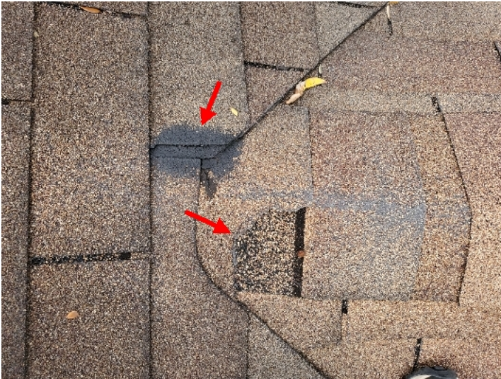
Damaged and torn ridge cap shingles.
