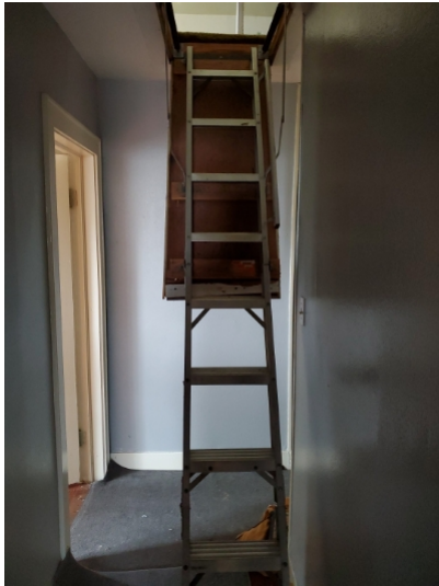
Damaged attic access ladder recommended repair/replace.
