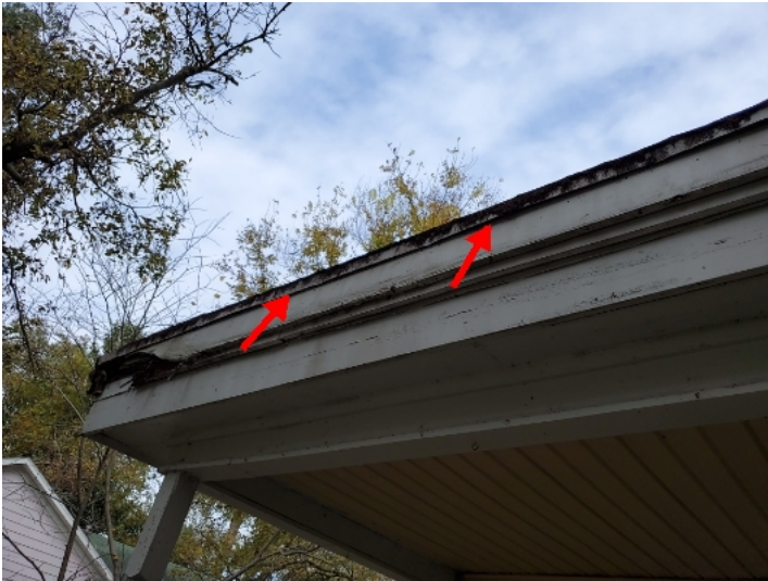
The roofing material on the front porch does not have the appropriate over hang on the left side causing water to drip down the fascia board on the front porch.
