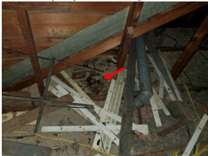
Damaged attic access ladder recommended repair/replace.
