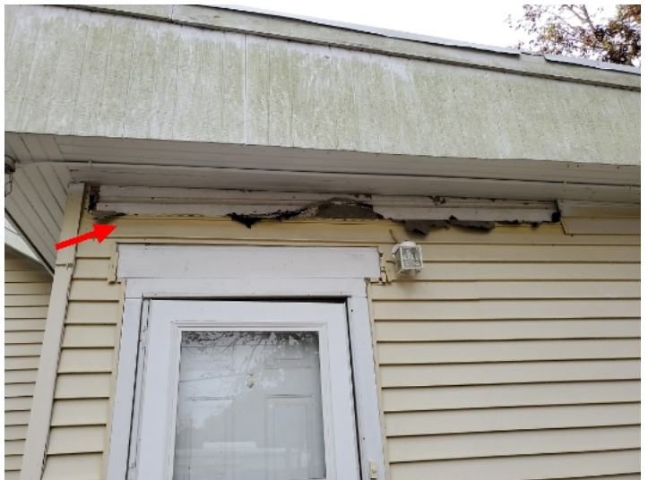
Section of missing vinyl siding of rear of house.
