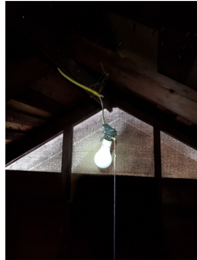
Open junction boxes and light fixtures that are not properly installed in attic.
