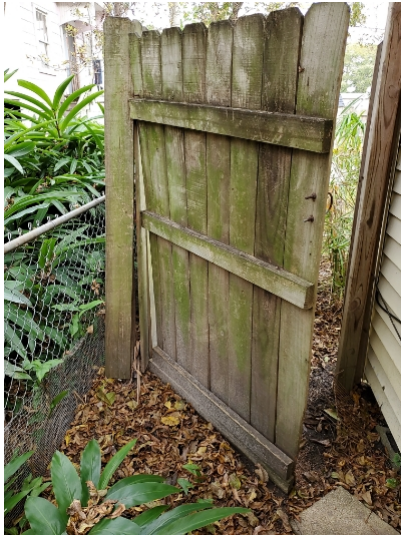
Left side gate is in need of adjustment and repairs.
