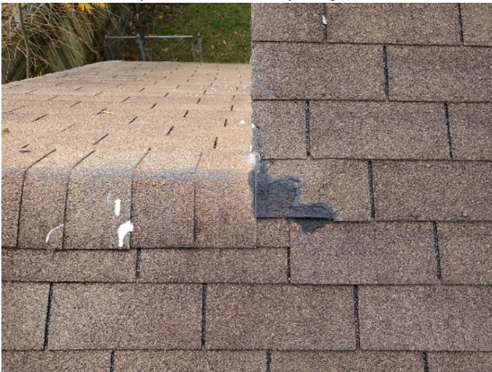
The roofing material on the front porch does not have the appropriate over hang on the left side causing water to drip down the fascia board on the front porch.
