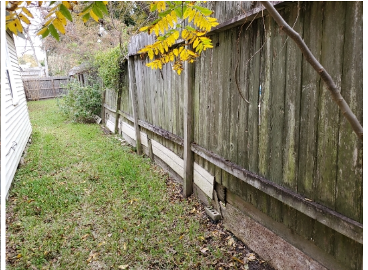
Various repairs to fence.
