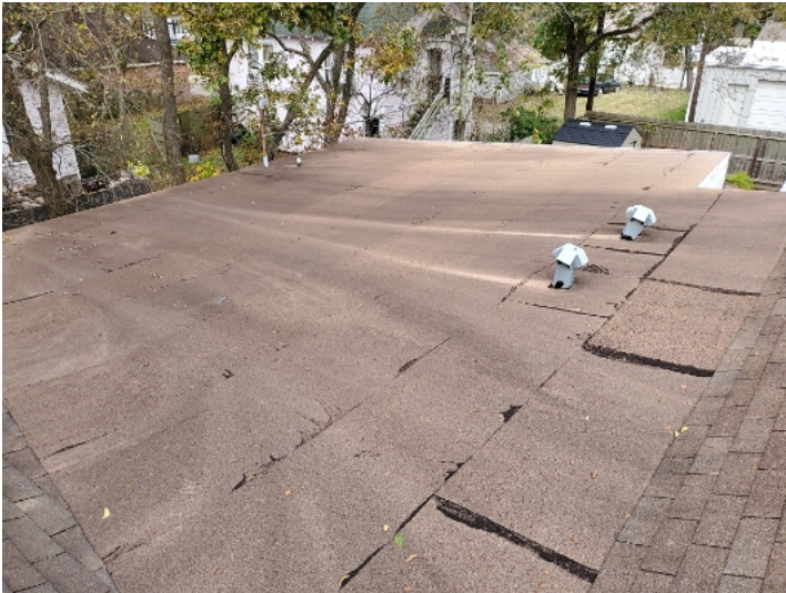
Damaged and torn ridge cap shingles.
