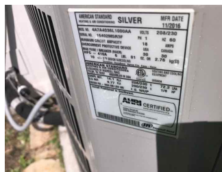
3 ton unit, made in 2016, uses 410a coolant, min/max amps: 18-30
