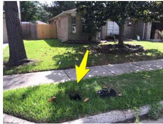
View of the water meter
