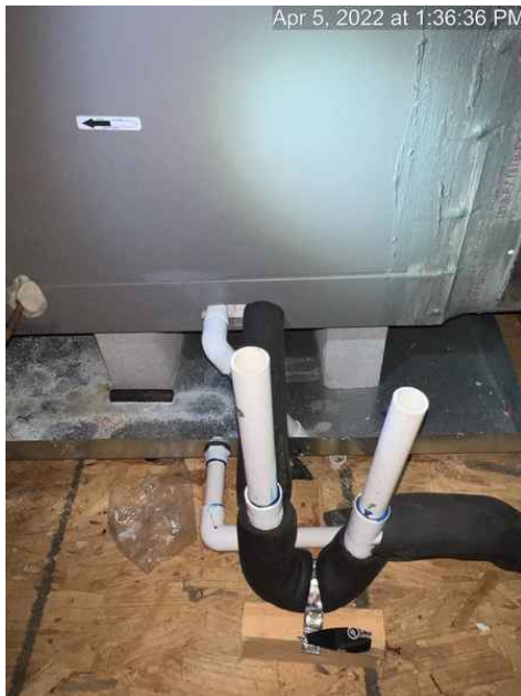
Typical condensate overflow switch
