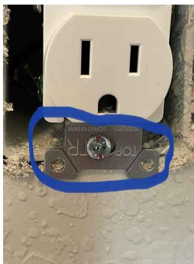
Sample of tamper resistant outlets
