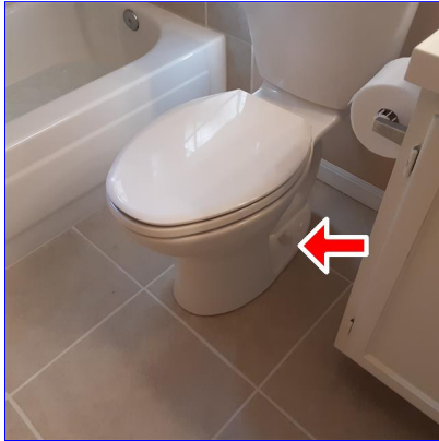
A. Item 3(Picture) 2nd floor guest bathroom
