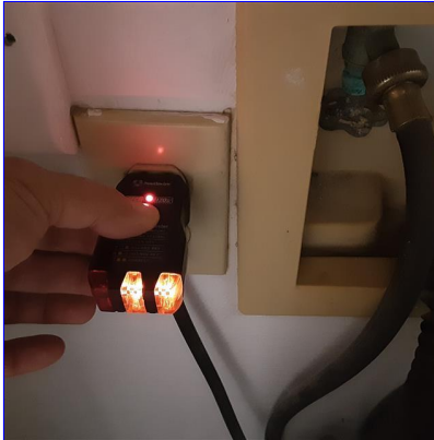
B. Item 2(Picture) Laundry room outlets
