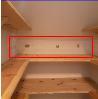
E. Item 1(Picture) Foyer closet
