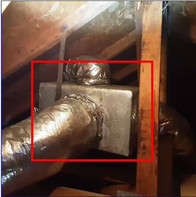
C. Item 1(Picture) In attic
