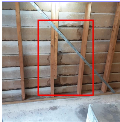
E. Item 10(Picture) Garage
