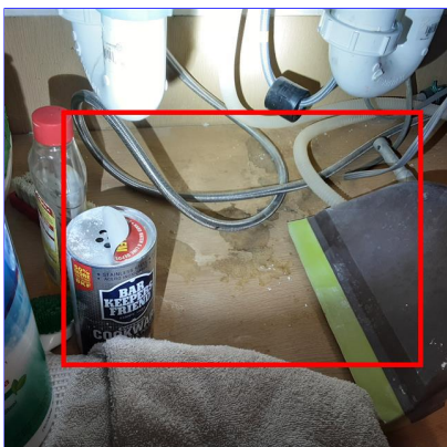
L. Item 1(Picture) Under kitchen sink
