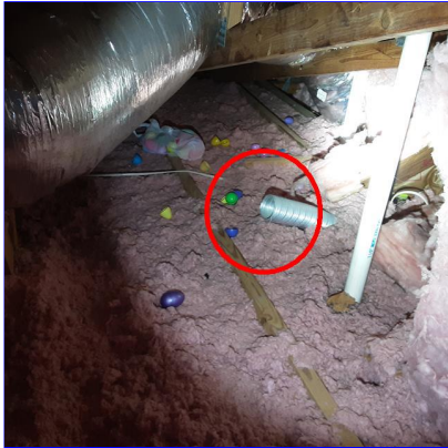
F. Item 1(Picture) In attic
