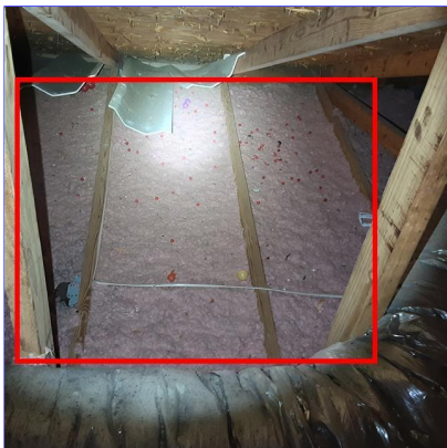
D. Item 4(Picture) Attic
