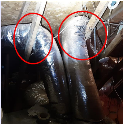
C. Item 2(Picture) In attic
