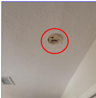
B. Item 8(Picture) 2nd floor hallway
