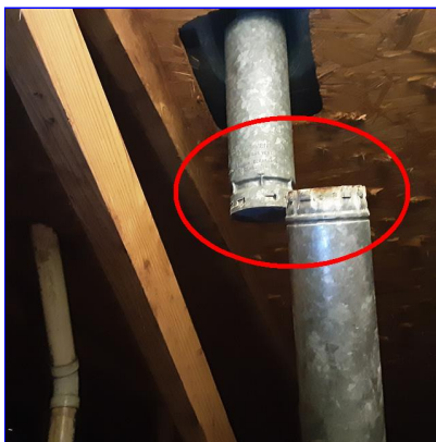
C. Item 5(Picture) In attic
