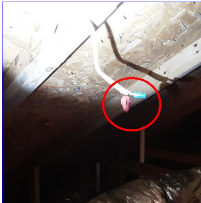
B. Item 13(Picture) Attic
