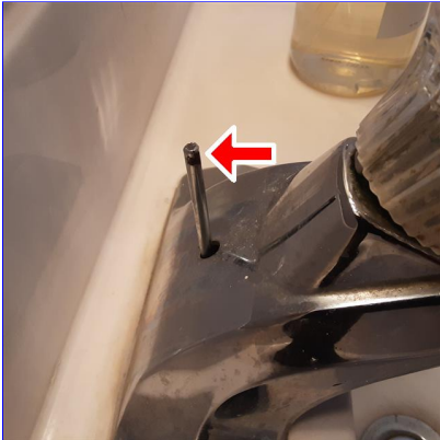
B. Item 1(Picture) 1st floor powder room
