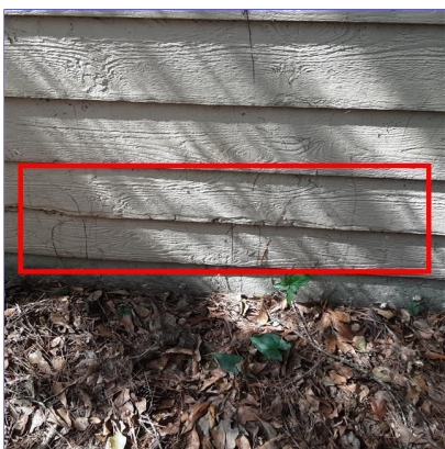
E. Item 6(Picture) Left side of garage
