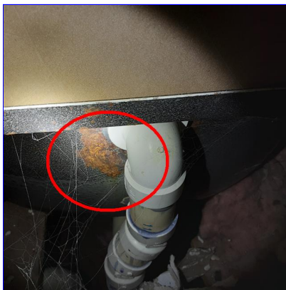
A. Item 5(Picture) 2nd floor guest bathroom tub
