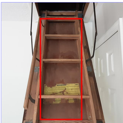
D. Item 2(Picture) Pull down stairs
