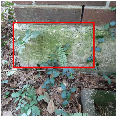
A. Item 1(Picture) Front right corner
