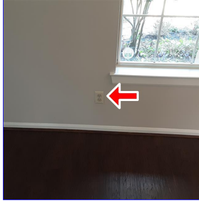
B. Item 5(Picture) Living room
