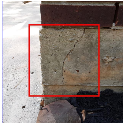
A. Item 2(Picture) Front left corner
