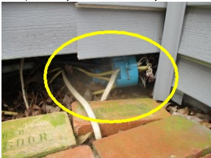
Open junction box with many exposed splices and exposed romex wire under home near breaker panel on right wall of home.
