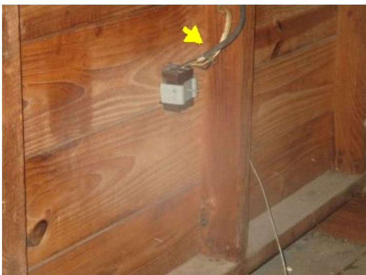
Exposed wire splices in attic areas are required be in protected junction box for safety reasons.
