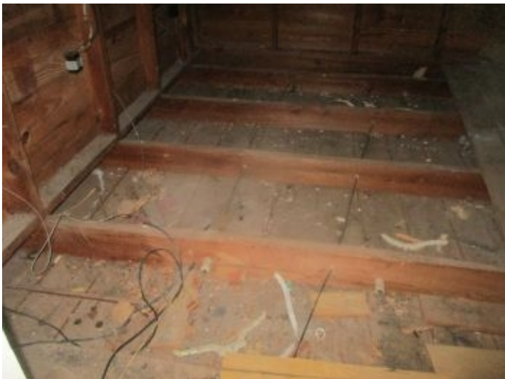
No attic floor and wall insulation observed in upper wall scuttle area.
