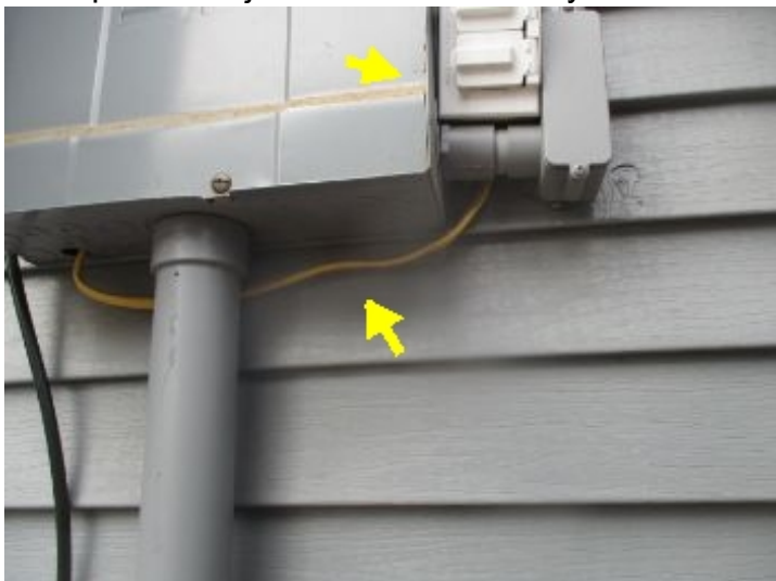
Loose exterior receptacle and exposed romex at exterior panel.
