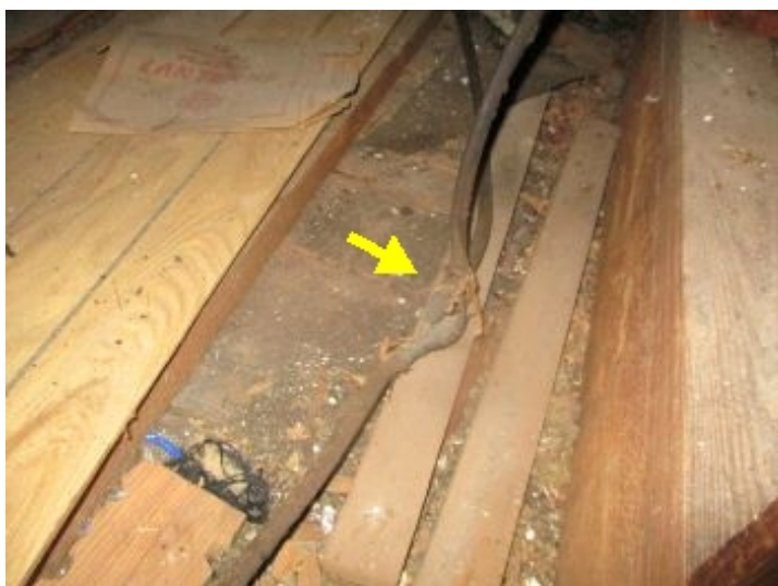
Exposed wire splices in attic areas are required be in protected junction box for safety reasons.
