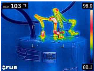
General Photos of Plumbing Fixtures:
