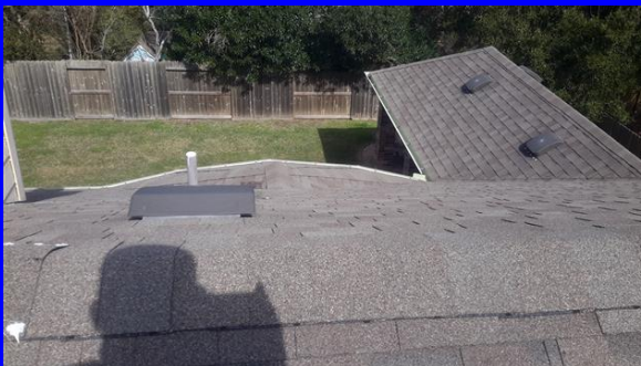
Roof overview, back
