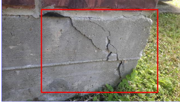
A. Item 1(Picture) Back corner near AC unit
