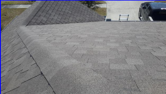
Roof overview, front
