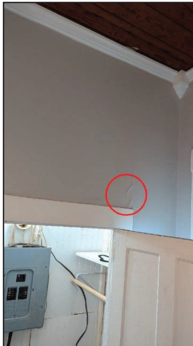
114. Poor joints
