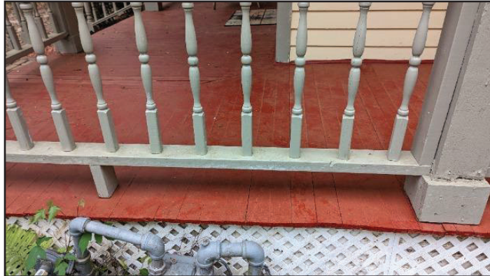
34. Spindles (balusters) climbable
