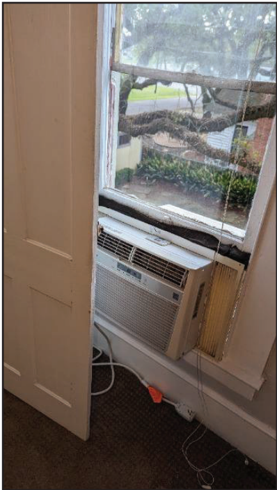
81. Window A/C excluded from inspection
