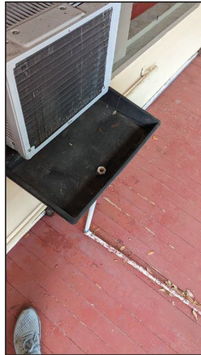
82. Window A/C excluded from inspection
