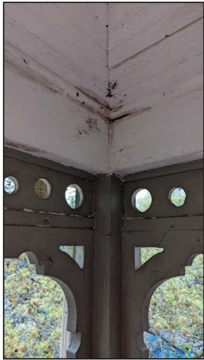
13. Rot or insect damage
