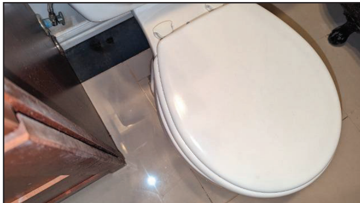
104. Floor damage suspected
