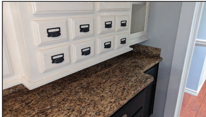
136. Pieces missing or loose
