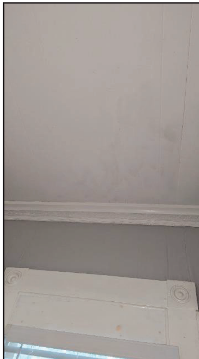
110. Water damage
