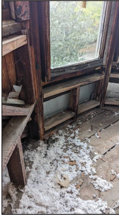
18. Water damage
