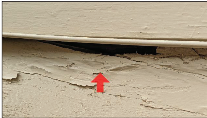
17. Rot or insect damage
