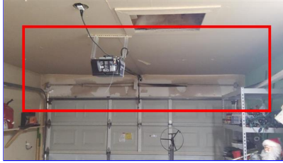
F. Item 5 (Picture) Garage
