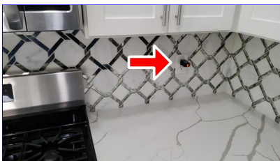
B. Item 9 (Picture) Kitchen
