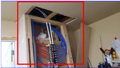
F. Item 1 (Picture) Garage
