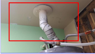
F. Item 4 (Picture) Garage
