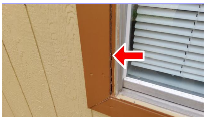
H. Item 3 (Picture) Left side
