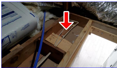
D. Item 3 (Picture) Attic
