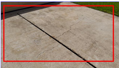
L. Item 5 (Picture) Driveway
