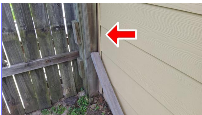
E. Item 21 (Picture) Right rear
