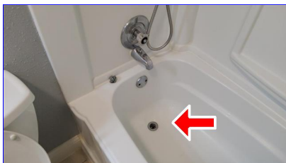
B. Item 1 (Picture) Hall bath
