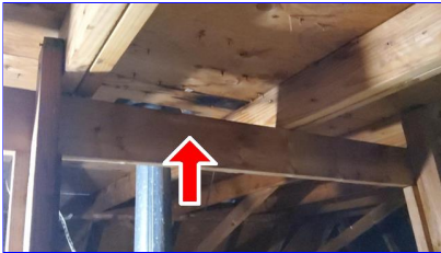
D. Item 7 (Picture) Near furnace vent
