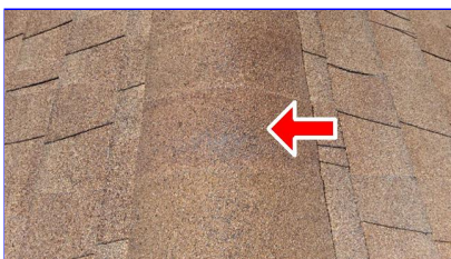
C. Item 3 (Picture) Roof
