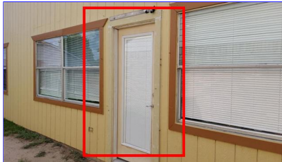
E. Item 14 (Picture) Side door trim
