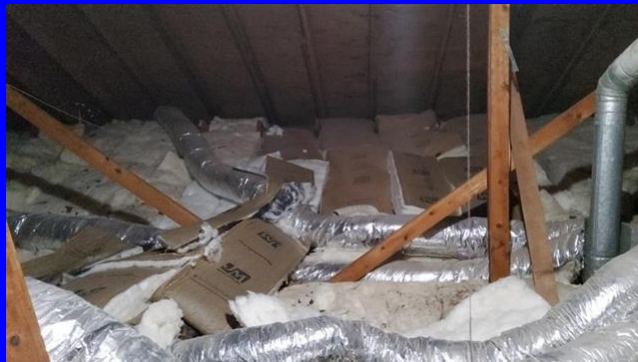
Batt insulation installed
