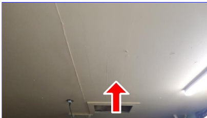
F. Item 2 (Picture) Garage
