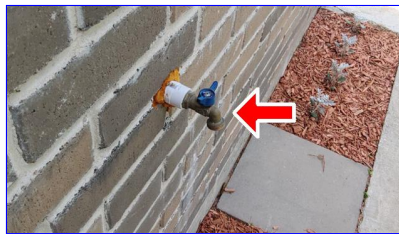
A. Item 2 (Picture) Exterior faucets
