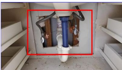
E. Item 27 (Picture) Hall bath
