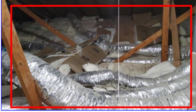
C. Item 2 (Picture) Attic
