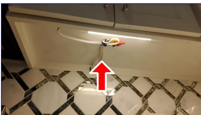
B. Item 14 (Picture) Kitchen
