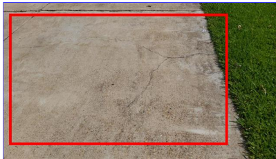
L. Item 4 (Picture) Driveway
