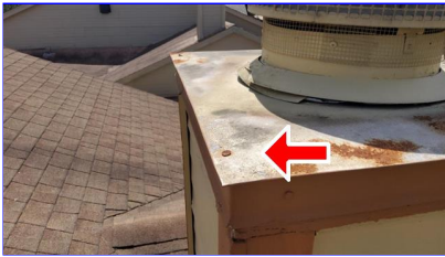
C. Item 7 (Picture) Chimney
