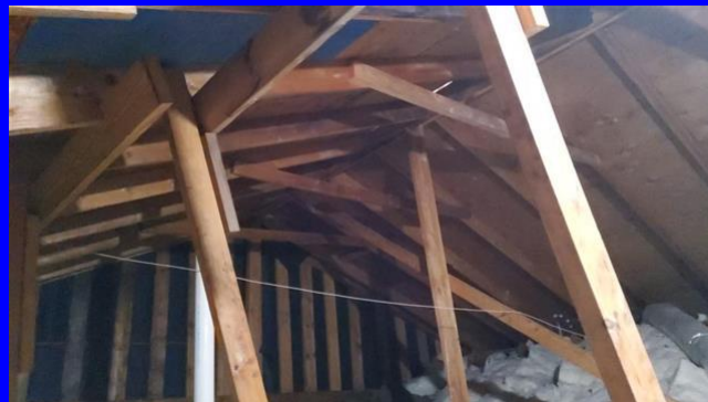
Roof structure stick built with plywood decking
