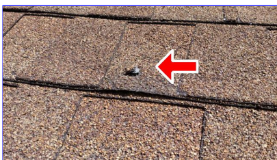
C. Item 4 (Picture) Roof
