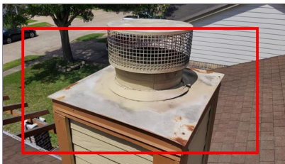
J. Item 1 (Picture) Chimney
