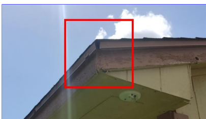
C. Item 2 (Picture) Left rear
