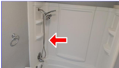
A. Item 3 (Picture) Shower wand can reach below bath water line
