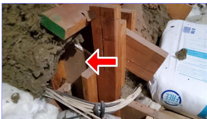
D. Item 4 (Picture) Attic
