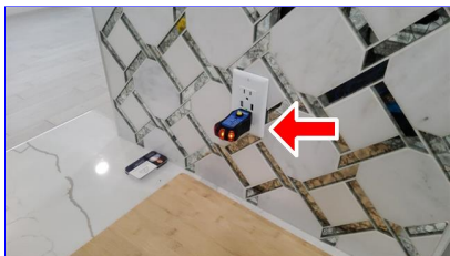
B. Item 6 (Picture) Kitchen
