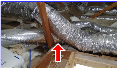
C. Item 3 (Picture) Attic
