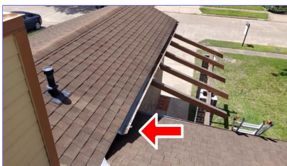
B. Item 8 (Picture) Gutters
