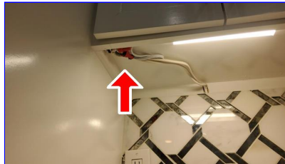
B. Item 13 (Picture) Kitchen
