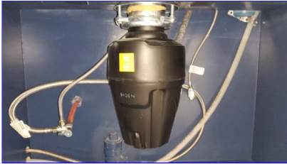
B. Item 1 (Picture) Kitchen
