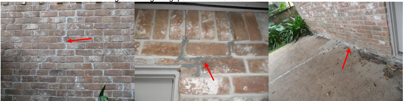
Brick mortar repairs
