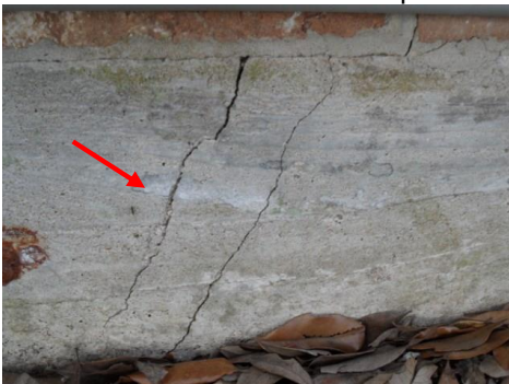
Foundation fracture
