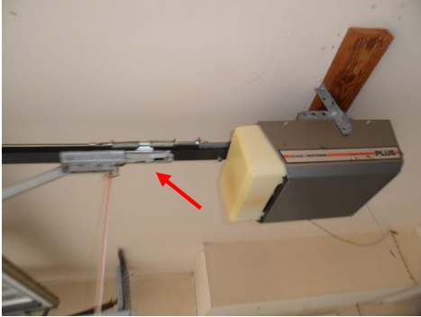
Trolley not engaged
