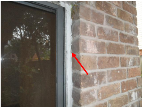
Calking repairs
