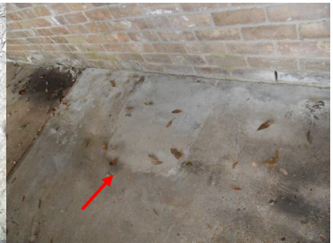
previous foundation repairs
