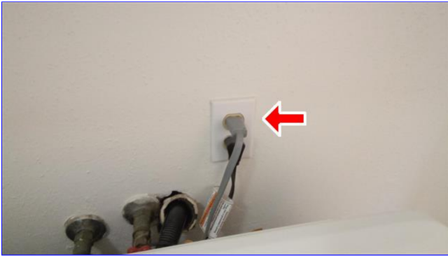
B. Item 2(Picture) laundry room
