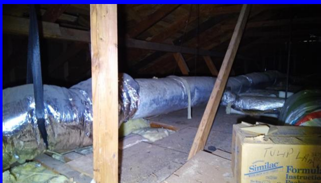
insulated ductwork
