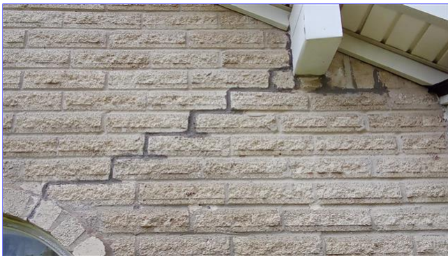
E. Item 4(Picture) front of home to right of main entry
