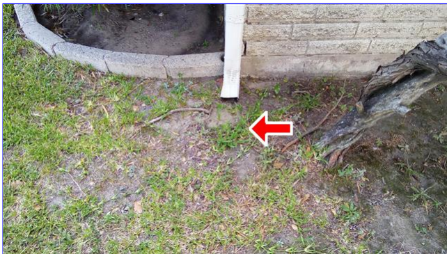
B. Item 1(Picture) at multiple locations
