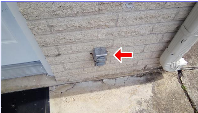
B. Item 4(Picture) exterior outlets
