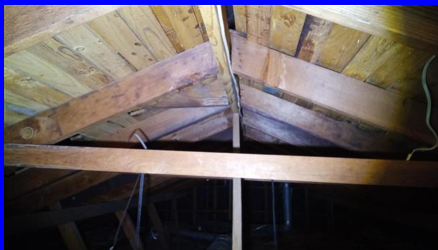
Stick built roof structure
