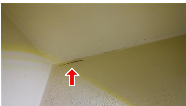
F. Item 1(Picture) top of master bedroom closet
