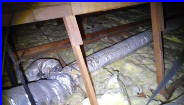
approximately 6 inches of insulation in the attic
