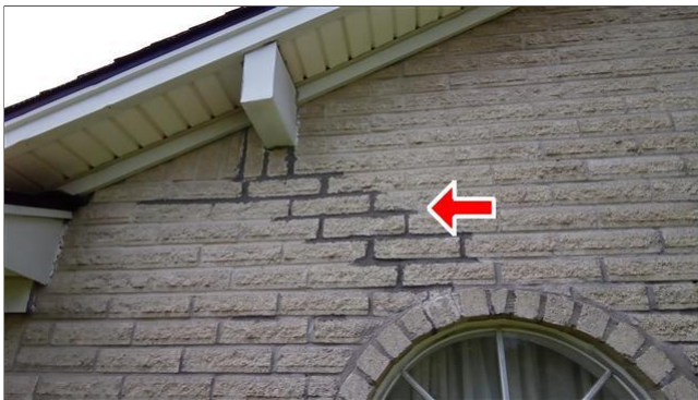
E. Item 6(Picture) front of home. left on main entry
