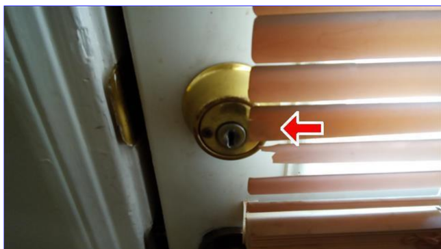
G. Item 2(Picture) laundry room exterior door
