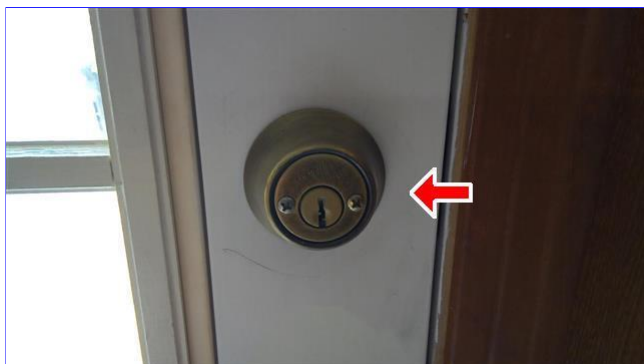
G. Item 1(Picture) rear living room door
