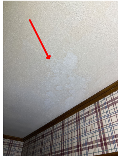
Moisture staining was noted on the ceiling of the garage above the water heater, the kitchen, the dining room. The cause for the staining should be determined, and repairs undertaken, if necessary, to prevent structural damage.
