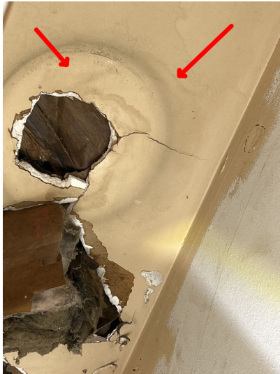
Moisture staining was noted on the ceiling of the garage above the water heater, the kitchen, the dining room. The cause for the staining should be determined, and repairs undertaken, if necessary, to prevent structural damage.
