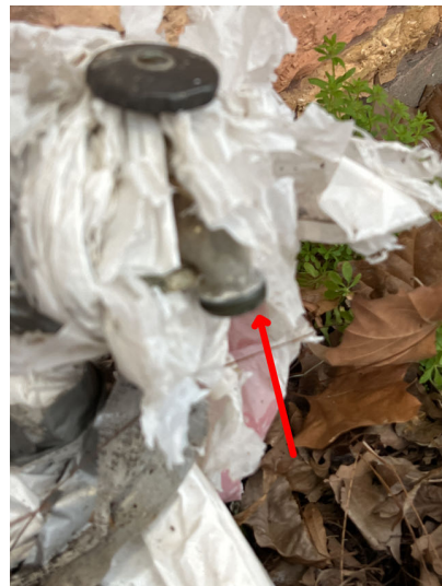
Even though the well is running, and the valves are open, no water pressure reaches the house.
