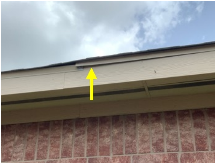
Lifting drip edge flashing on the left side of this home.
