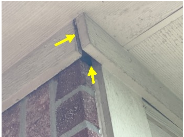
Gap between the brick and brick frieze on the right rear corner of this home.
