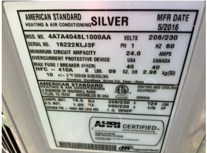
Condensing unit data plate.
