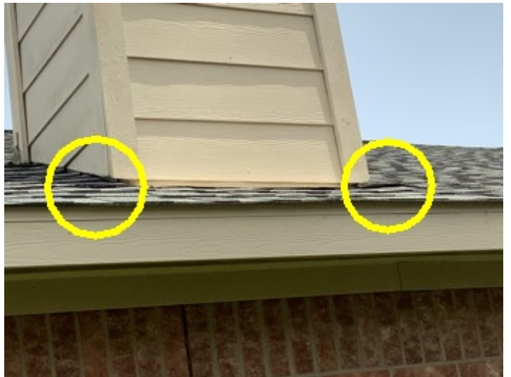
Lifting step and counter flashing at the chimney.
