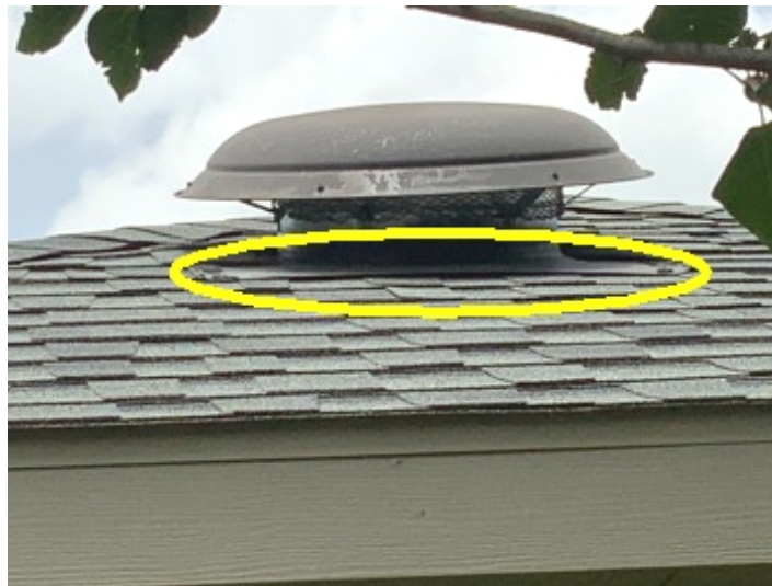
Lifting attic vent cover flashing on the rear of this home.
