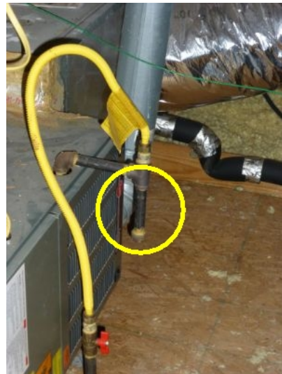
Example of a gas pipe sediment trap.
