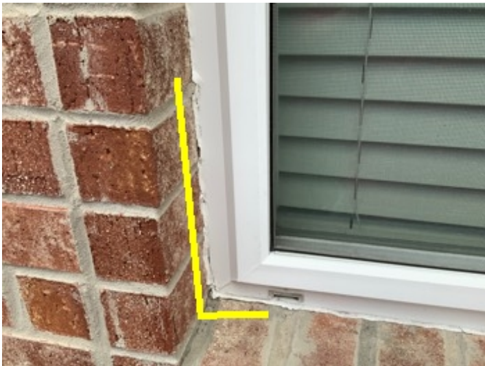
Sealant gaps at the rear window on the left side of this home.
