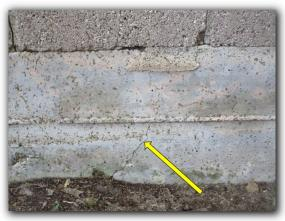
There is exposed aggregate with exposed plumbing at the rear of the home near the rear left corner.
