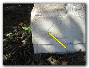
There are large trees in close proximity to the foundation. I recommend monitoring this area of the home for any signs of movement. Underground roots can cause slab movement.
