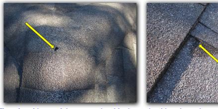
There is evidence of damage to the shingles at the ridge above the rear left corner of the home.
