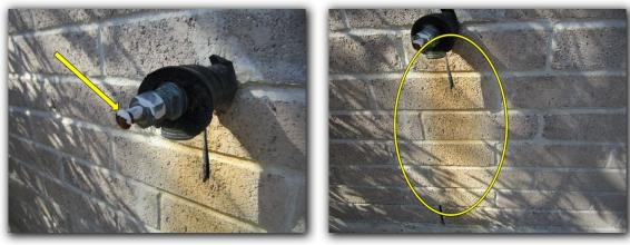
The main water supply line is not fully / properly insulated, with evidence of a leak at the main line.
