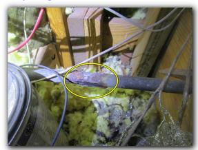
There is evidence of corrosion on the water supply lines in the attic above the hall with signs of prior repair to the supply lines at more than one location.
