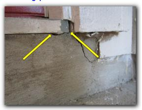
There is a mortar joint crack with loose bricks at the top front right corner of the garage.
