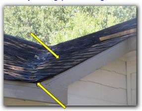
There are roof jacks that are damaged and need to be replaced at more than one location on the roof.
