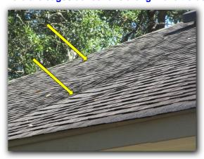
There is extensive damage to the roof at the rear of the home above the rear right bedroom and master bathroom areas.
