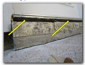
There is evidence of rotting wood at the base of the trim at the rear right corner and at the rear entry door trim.
