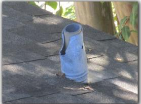
The rain collar is not fully / properly seated on the vent pipe.
