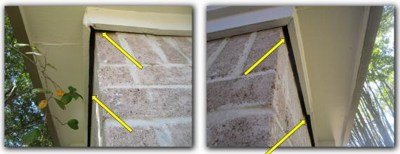
There is deteriorated caulking material at the brick / trim intersection at the kitchen box window frame trim.
