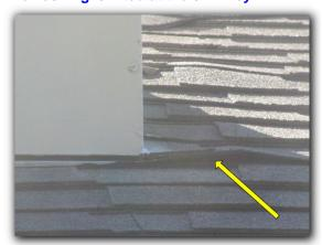
There are exposed nail heads on the roof. Nail heads should be sealed with roof caulking material. Over time, water may penetrate the roof around a rusted nail if they are not properly sealed.
