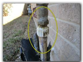
Due to the age of the home, the galvanized plumbing and the signs of foundation movement, I recommend a complete review of the plumbing system, including scoping the underground lines for any damage, leaks or other deficiencies by a licensed plumber. I recommend asking the seller if the underground plumbing has already been reviewed / scoped (including any optional hydrostatic pressure test). If so, ask for a copy of the report.
