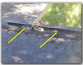
The shingles are showing signs of age with damage and wear, including loss of granular material.
