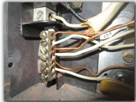
The color of branch circuit wires are required to be black, red, or marked. There are white branch circuit wires that have not been marked as required.
