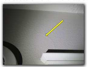
NOTE: There are signs of prior repair to the interior walls throughout the home, including sheet rock, texture, and paint. This may conceal prior signs of damage or foundation movement.
