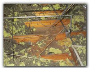
There is a required minimum 24" wide, unobstructed walkway to all attic equipment. The walkway is obstructed / inadequate, creating a potential trip hazard.
