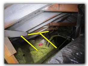
There is no palm bracing where the rafters meet the end of the ridge beam.
