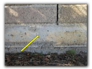
There is exposed aggregate on the left side of the home near the main water supply line.
