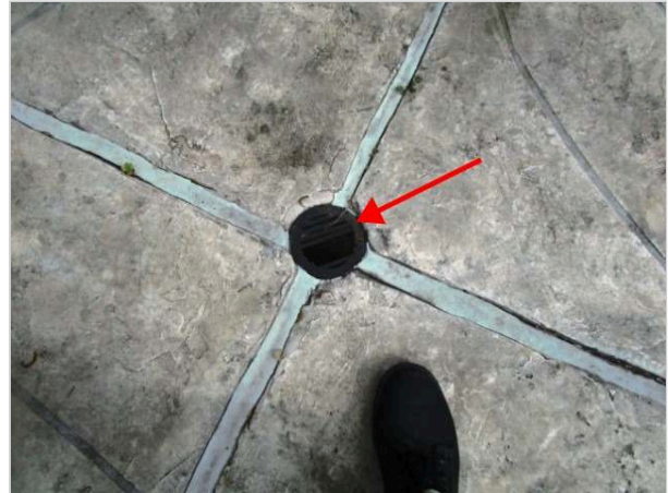
Damaged grate
