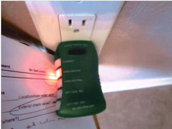
Indication of open ground - kitchenette rear wall
