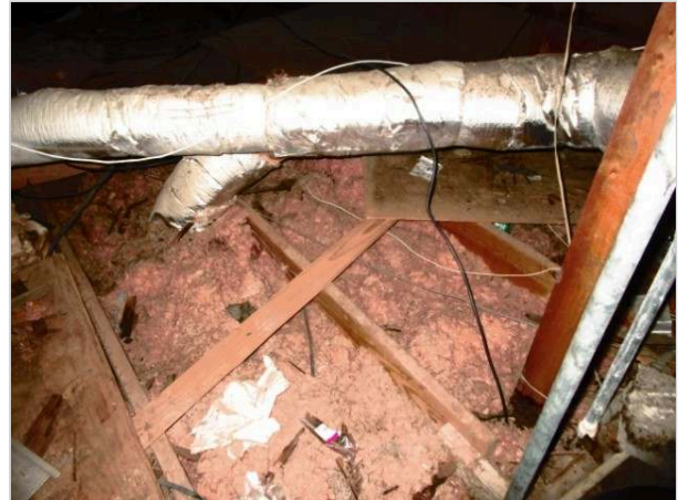
Attic view - compressed blown insulation
