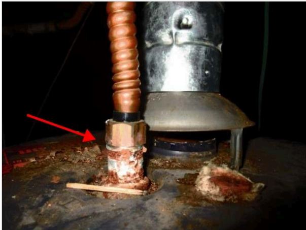
Rusted / corroded
