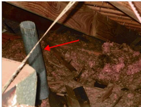
Terminating in attic
