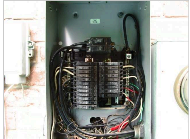
Cover removed for inspection.
