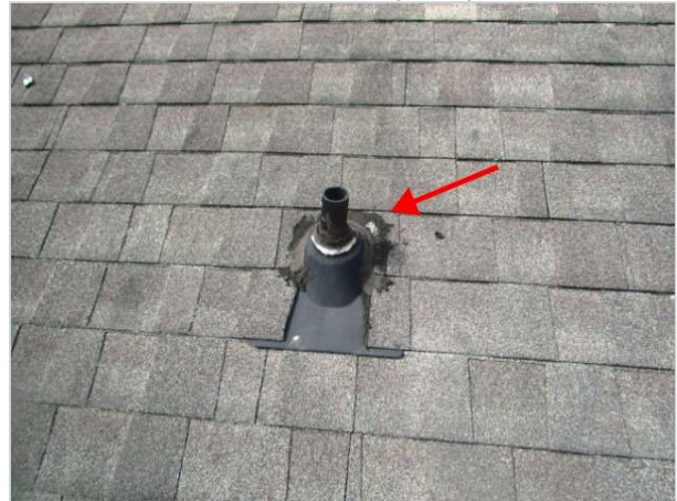
Roofing tar used around boot jacks
