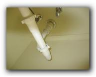
24. Observed leaking drain under upstairs bathroom sink. These leaks can promote water penetration to the structure. Concealed damage is a possibility. Recommend having a licensed plumber repair the issue.
