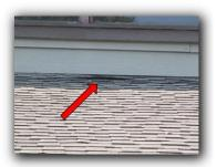
Observed various nails backing out of roofing material.
