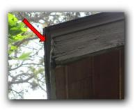
6. Wood decay (water damage) was detected on the surrounding deck, porch or balcony. Weathered lumber should be treated with a water proofing product. This oil based products can be purchased at most home improvement stores and are easy to apply. Water damaged elements should be replaced or repaired. This condition can also be conducive to insect infestation. Timbor is another product to protect exterior decking from various types of wood destroying organisms.
