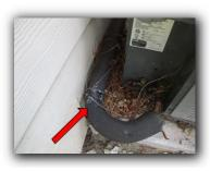
21. Observed missing protection cover for exterior piping material.
