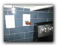
17. Ground Fault Interrupter outlets would not reset, outlets dead:
