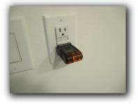
16. GFCI (ground fault circuit interrupter) not tripping when tested with external device in upstairs bathroom
