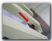
7. Observed loose balusters. Recommend repair to prevent possible injury.
