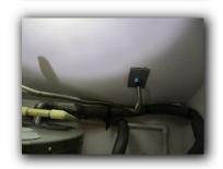
28. No electric service disconnect installed at unit.
