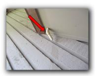
26. Temperature & Pressure relief valve (TPR) should drain into a line that is plumbed horizontally or down, but cannot go back up (this keeps debris from going back to the valve). This line can be 3/4 inch C.P.V.C. plastic (not reduced in size) and should terminate from 6 to 24 inches from the exterior ground with an elbow facing down. Remember to test the valve and replace it if it leaks or does not operate or every 3 years.
