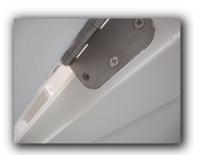
3. Hinge screws missing various locations. The hinge screws serve two purposes in the function of an exterior door. First they all need to be installed for security purposes, and second the weight of an exterior door is that which requires extra support.
