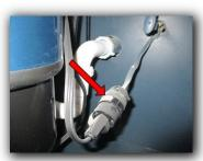
19. Extension cords are being used as permanent wiring under kitchen sink. Using extension cords as permanent wiring poses a fire and shock hazard, and is an indication that wiring is not adequate and should be updated. Recommend having a qualified electrician evaluate and make modifications as necessary. See UL reference on extension cord label.
