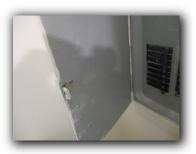
10. The circuit breakers are not identified and labeled. Proper labeling of circuit breakers can be crucial during an emergency situation.
