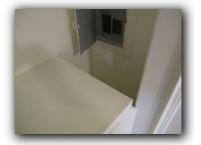
9. Proper working space is not provided at the front of the panel. A minimum of 3 feet in front of panel by 30 inches wide by 6 feet 6 inches.
