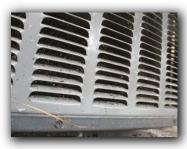
22. Condenser leaves or debris on it. Recommend cleaning this area so it can function properly.
