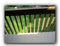
Spacing of posts on balusters and banisters that are higher than 30 inches above grade is changing in the industry. 5. The spacing of these posts should not exceed "4" inches. Because it is a safety concern with regard to small children, T.R.E.C. guidelines require that it be pointed out in this section of the report.
