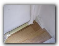
27. Observed TPR valve drain line is connected directly to safety pan drain line. Recommend having a plumber install a check (one way) valve between the safety pan and TPR drain line. This will help prevent possible water from entering the safety pan if the TPR valve was to open.
