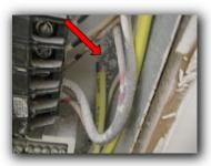
11. Wires were improperly spliced or terminated. Wire ends or splices should be capped or in junction boxes that are properly mounted. This condition is considered an electrocution/fire hazard and should be serviced by a licensed electrician.
