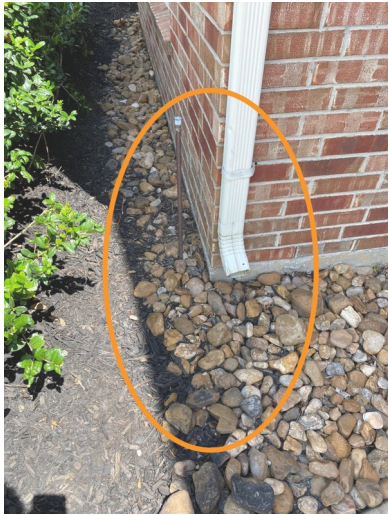
Example Front Exterior Wall
