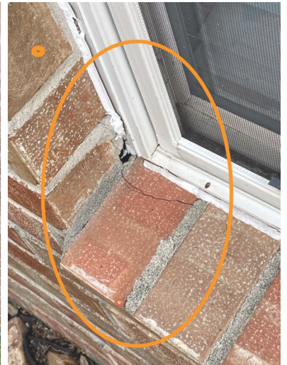
Example Front Exterior Wall
