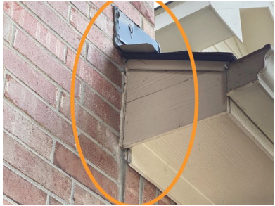
Example Front Exterior Wall
