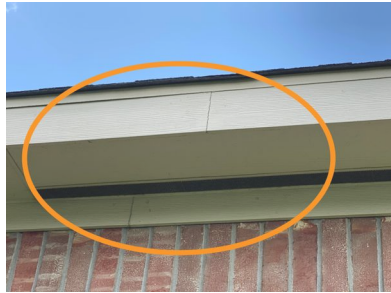
Example Rear Exterior Wall
