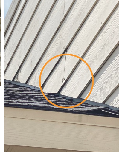
Example Rear Exterior Wall
