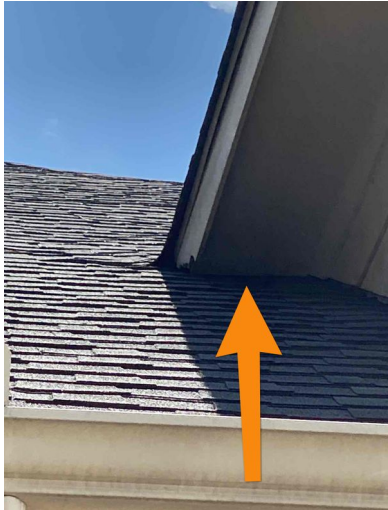
Example Front Exterior Wall
