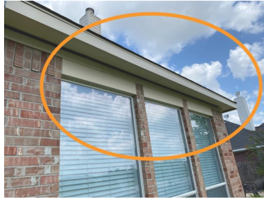
Garage Rear Exterior Wall
