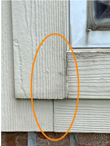
Example Rear Exterior Wall
