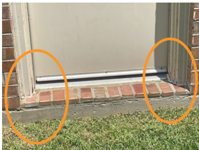
Example Right Exterior Wall
