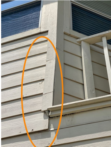
Example Example Rear Exterior Wall
