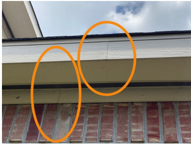
Example Right Exterior Wall
