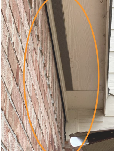
Example Rear Exterior Wall
