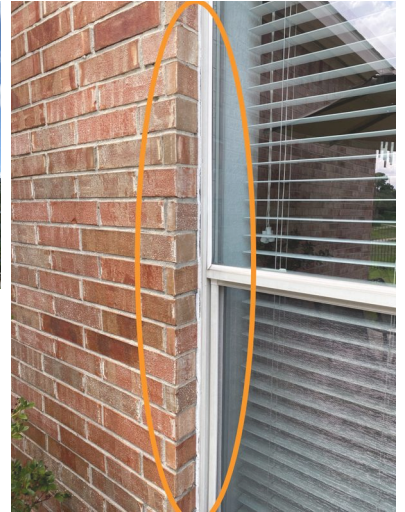
Example Rear Exterior Wall
