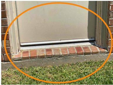
Example Right Exterior Wall
