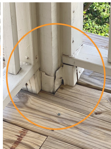
Example 2nd Floor Balcony
