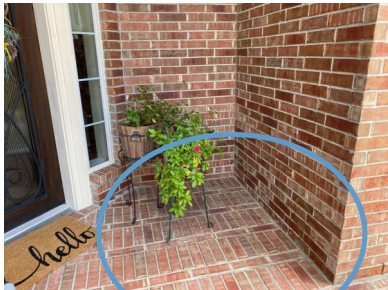
Example Front Exterior Wall
