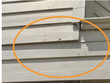
Example Rear Exterior Wall
