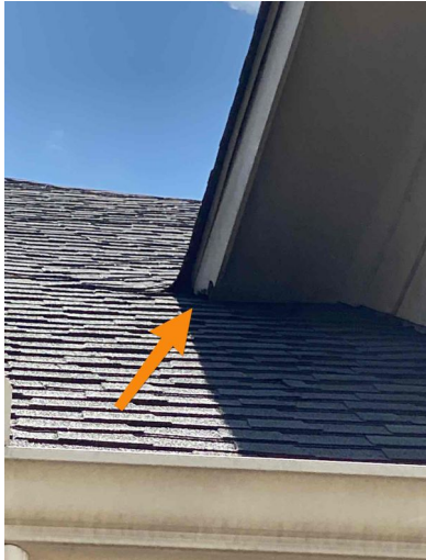
Example Front Exterior Wall
