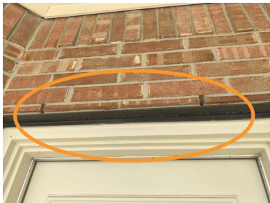
Example Rear Exterior Wall
