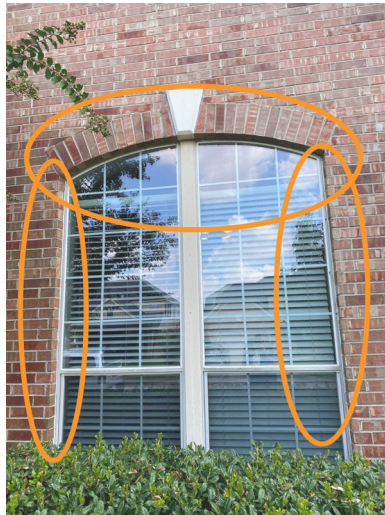
Example Front Exterior Wall
