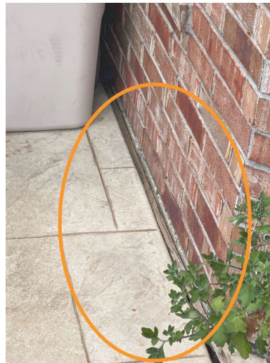
Example Rear Exterior Wall
