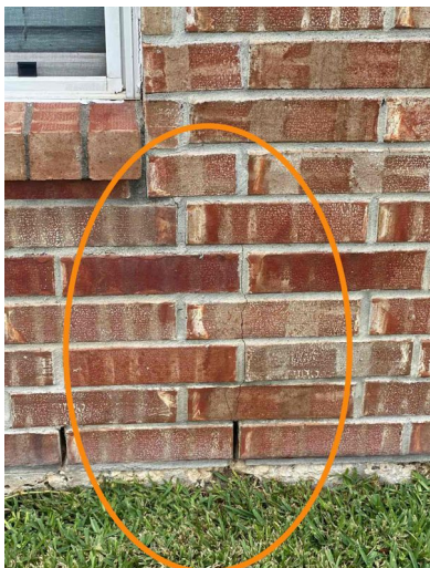
Example Rear Exterior Wall
