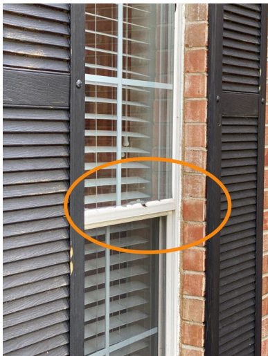
Example Front Exterior Wall
