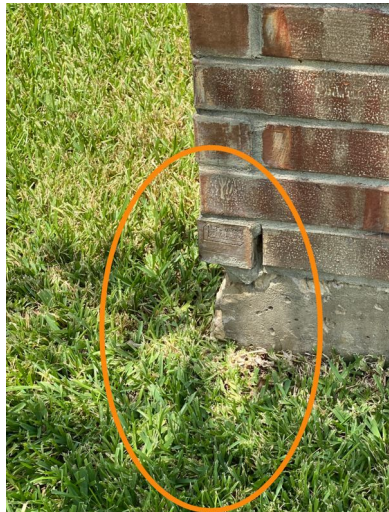
Example Rear Exterior Wall
