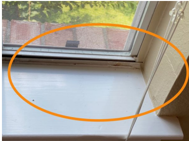
Example 2nd Floor Front Exterior Wall
