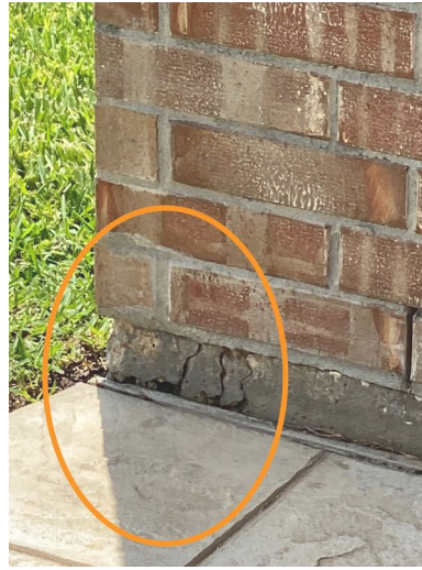
Example Rear Exterior Wall
