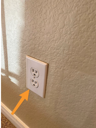
2nd Floor inside balcony
