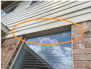
Example Rear Exterior Wall
