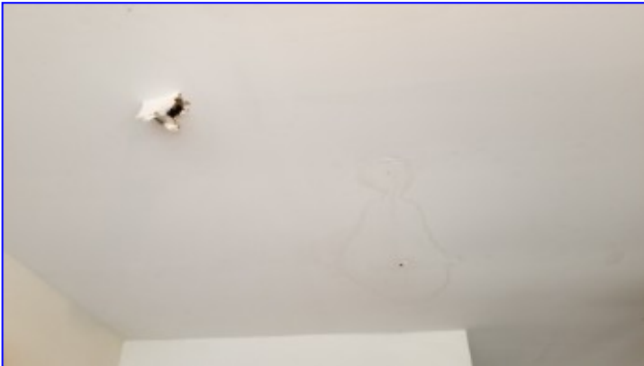
Water staining was observed in the garage. The cause/source should be determined and repairs undertaken, if necessary, to prevent further damage. Area dry at this time.
