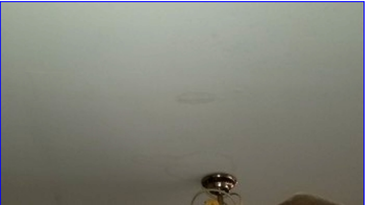
Water staining was observed in the garage. The cause/source should be determined and repairs undertaken, if necessary, to prevent further damage. Area dry at this time.
