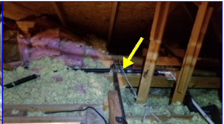
The primary condensate drain lines are tied together. This is not an ideal installation because if the line becomes obstructed, then both units are backed up. Recommend separating lines so that each unit is served by separate drain lines.
