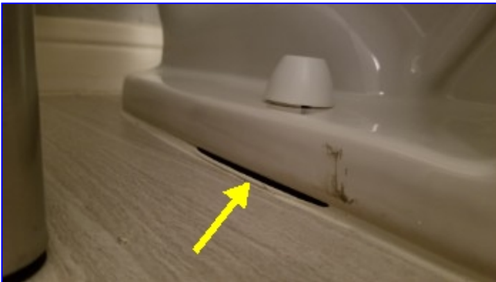
The commode in the right hand guest bathroom is not properly sealed at the floor. Improvements recommended to prevent the potential for sewer gasses entering the home.
