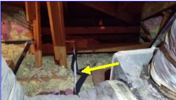
Missing insulation on primary condensate lines should be repaired/replaced to prevent moisture damage to the adjacent materials.
