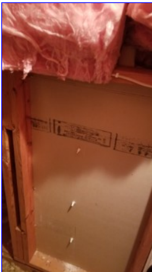
Loose batting was observed in the right rear attic space. This area should be improved/repared to ensure a proper thermal boundary is maintained.
