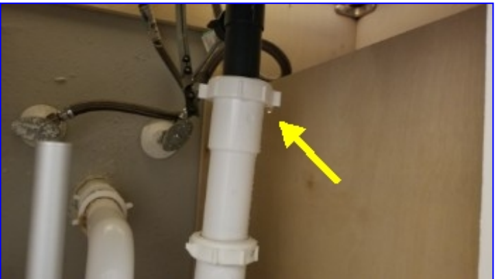
A leak was observed at the drain pipe connection under the left hand master sink. Repair recommended to prevent damage to the adjacent materials.
