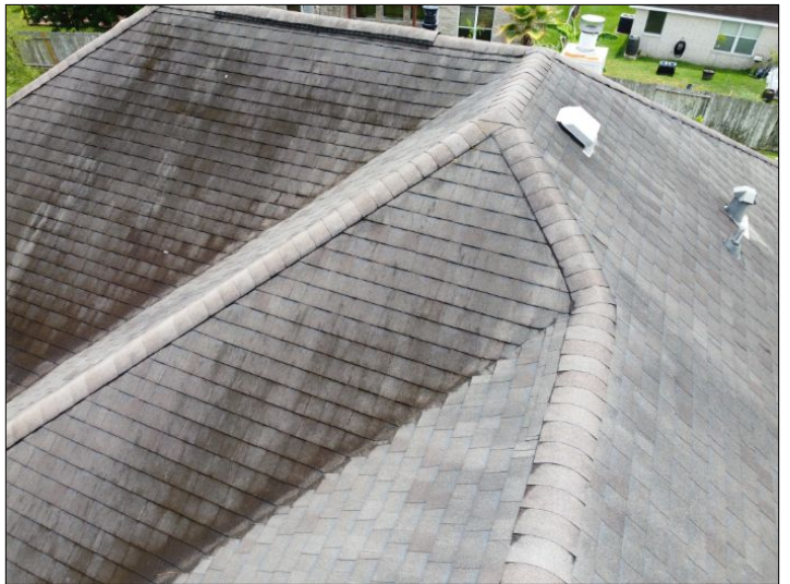
Overview of roof
