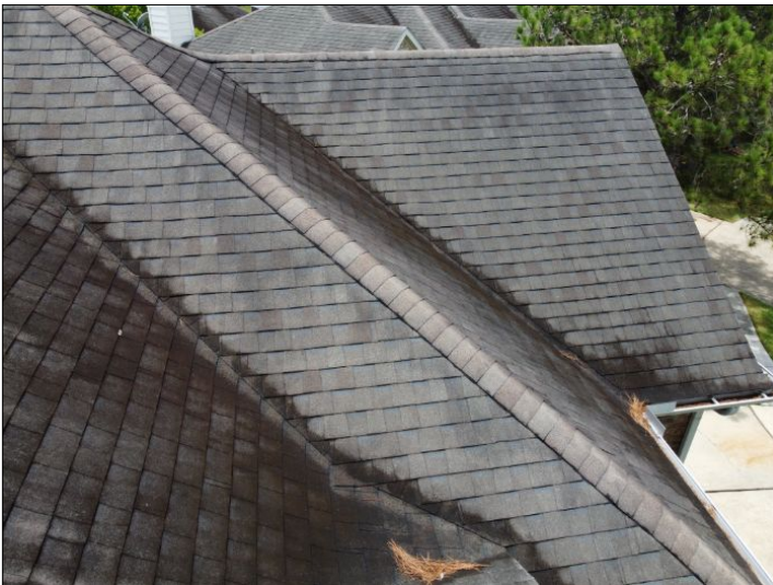
Overview of roof
