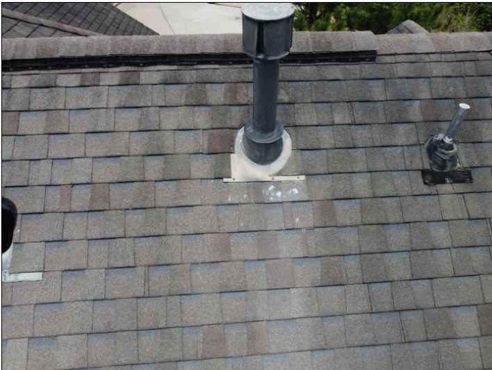
Overview of roof
