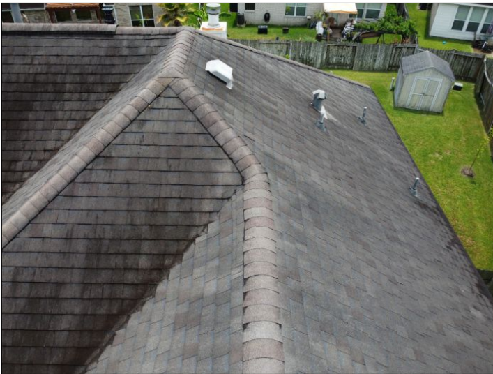
Overview of roof
