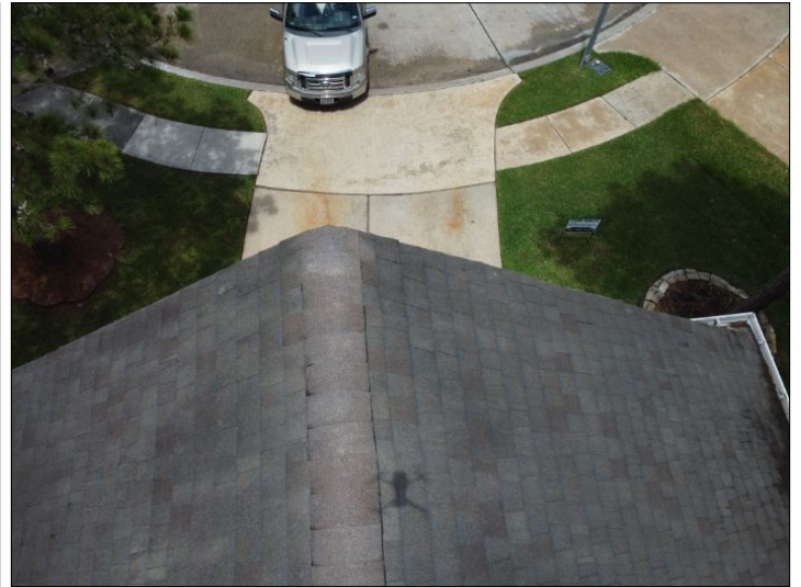
Overview of roof
