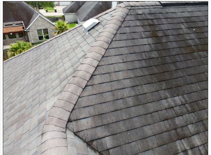
Overview of roof
