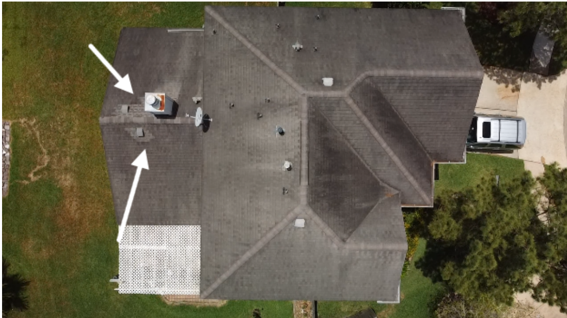
Previous Repair locations. No damaged, broken or missing shingles.
