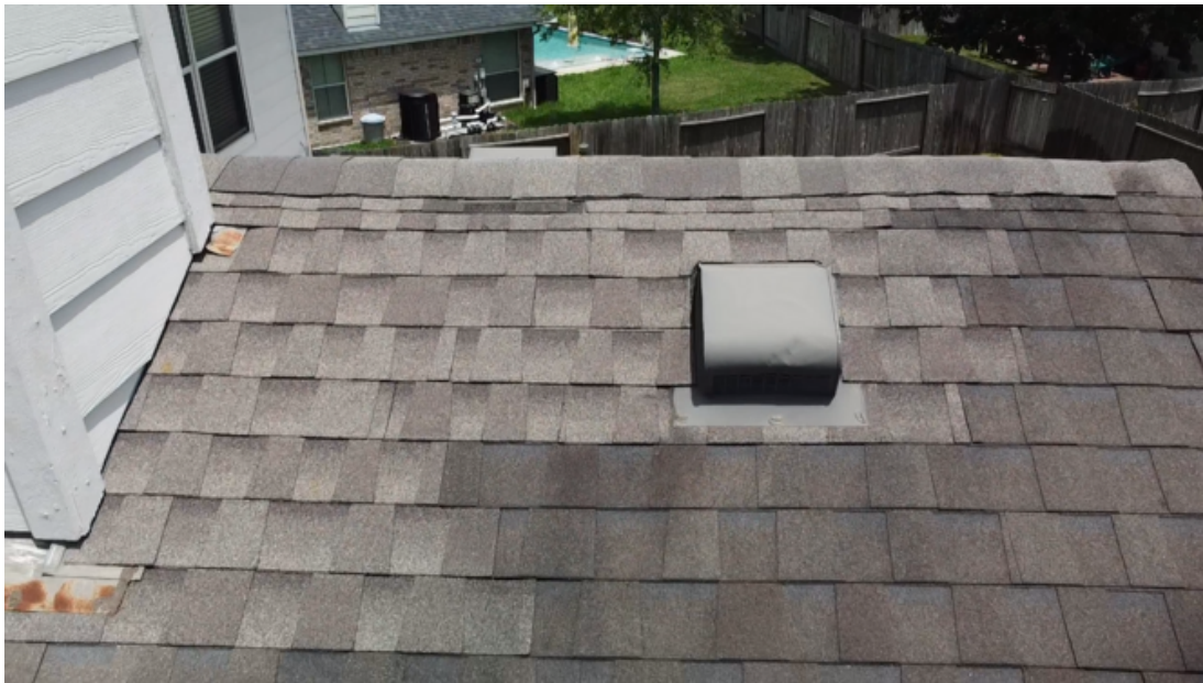
Previous repair and vent replacement.
