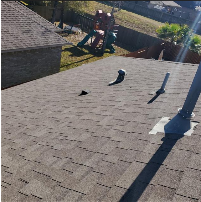
C. Item 3(Picture) Roof overview.
