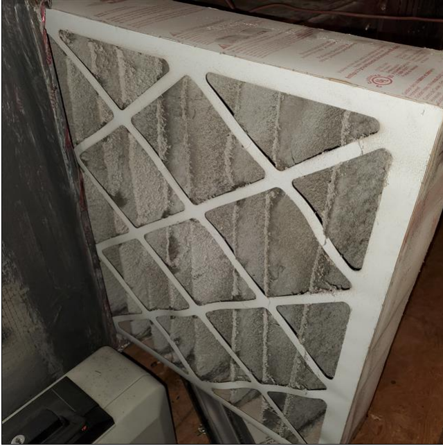
C. Item 3(Picture) Photo of dirty air filter.
