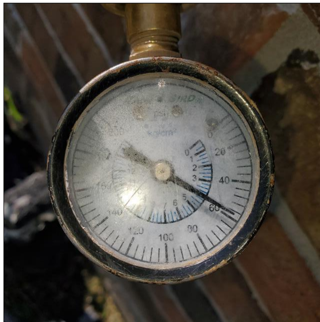
Water pressure was 58 psi (acceptable)
