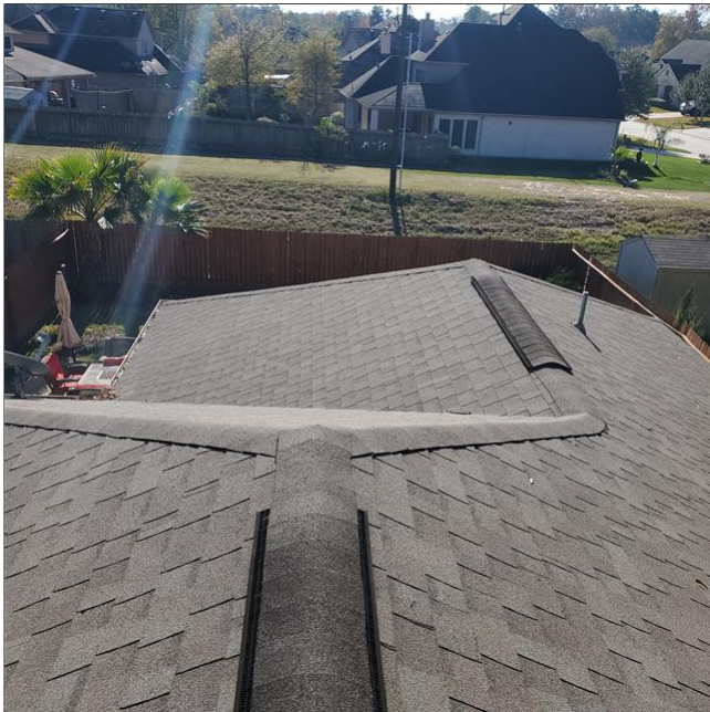
C. Item 4(Picture) Roof overview.
