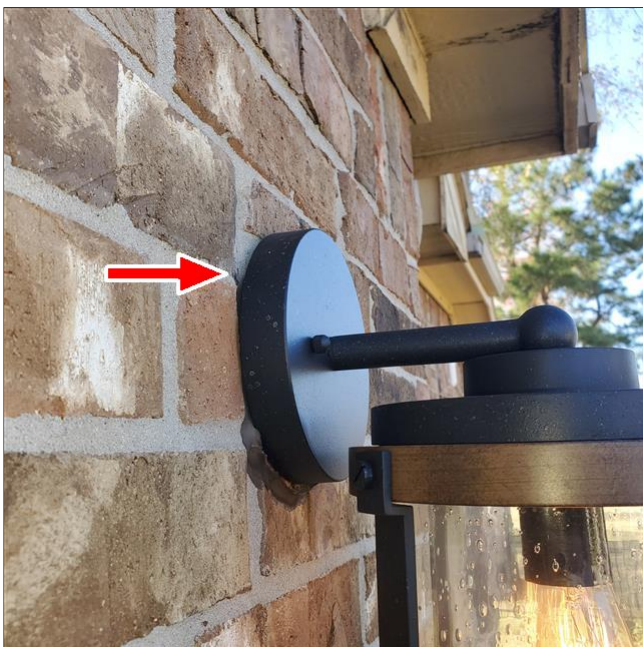
E. Item 1(Picture) Need to seal all light fixtures to the wall.
