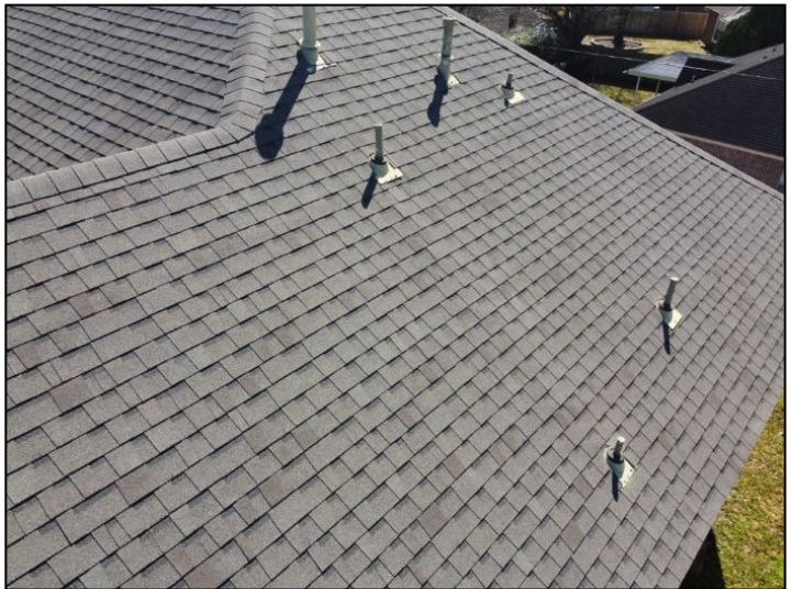
ROOF COVERING; RIGHT
