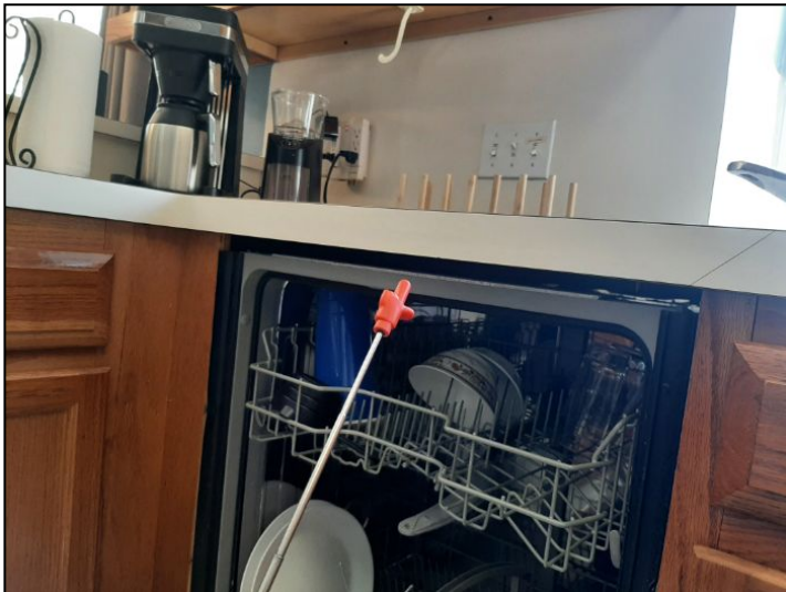
LOOSE / UNSECURED APPLIANCE
