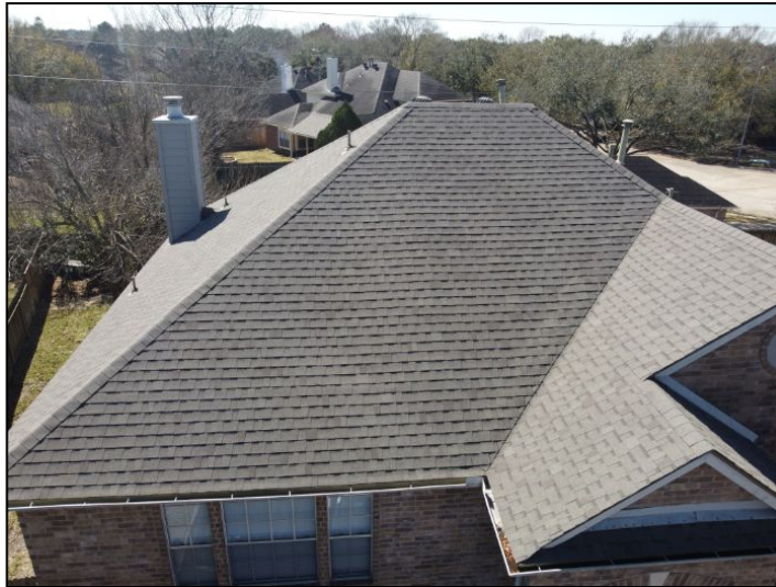
ROOF COVERING; FRONT
