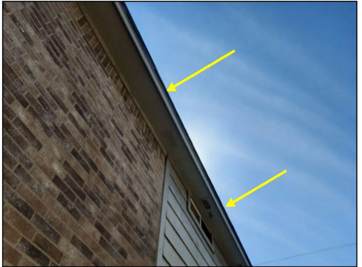
NO GUTTER SECTIONS
