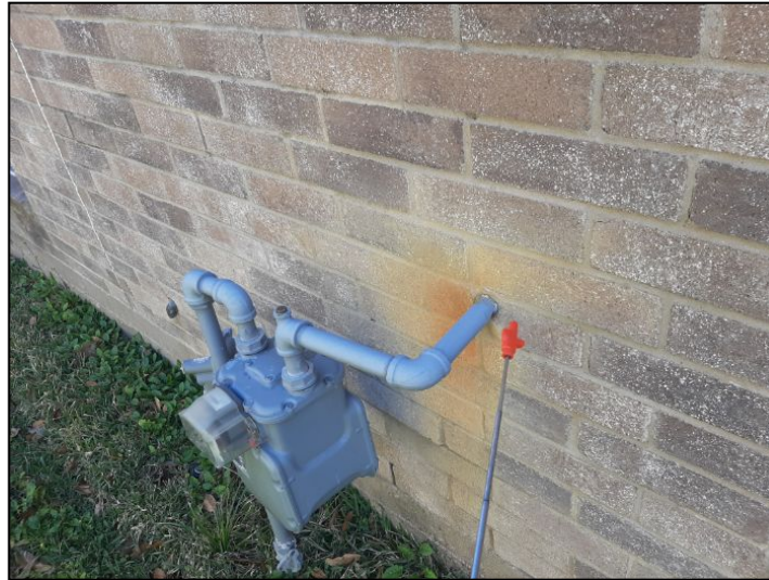
MISSING BONDING
