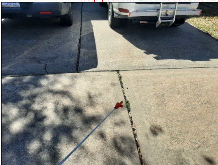
EXPANSION DETERIORATION
