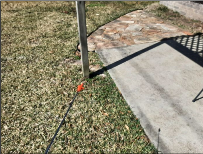
POST IN CONTACT WITH SOIL
