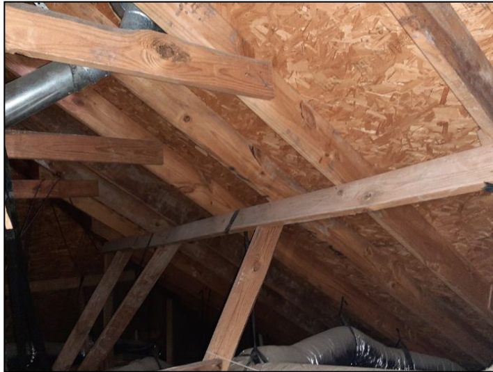
ATTIC STRUCTURE OK; NO RADIANT BARRIER
