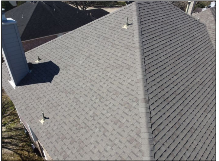
ROOF COVERING; LEFT
