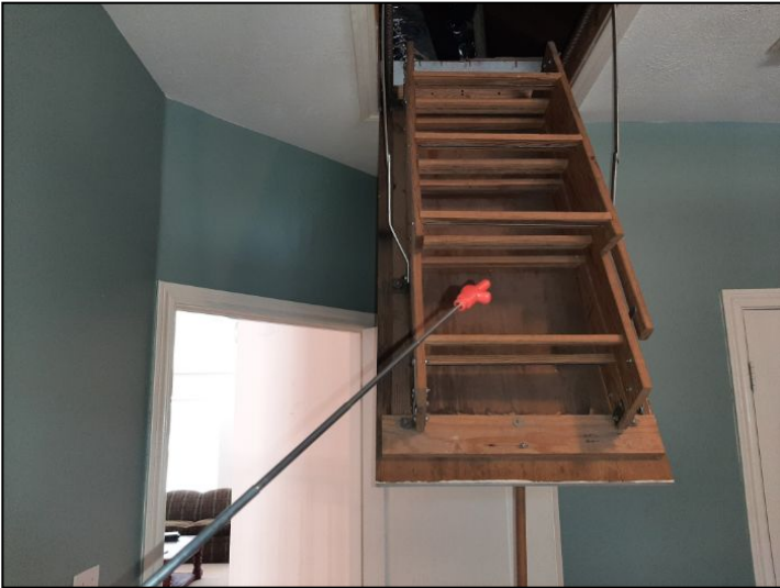
MISSING INSULATION
