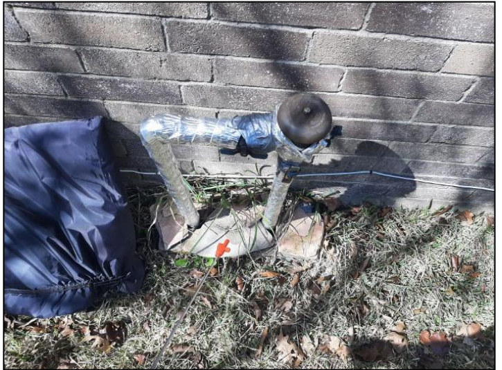
INSULATION DETERIORATION
