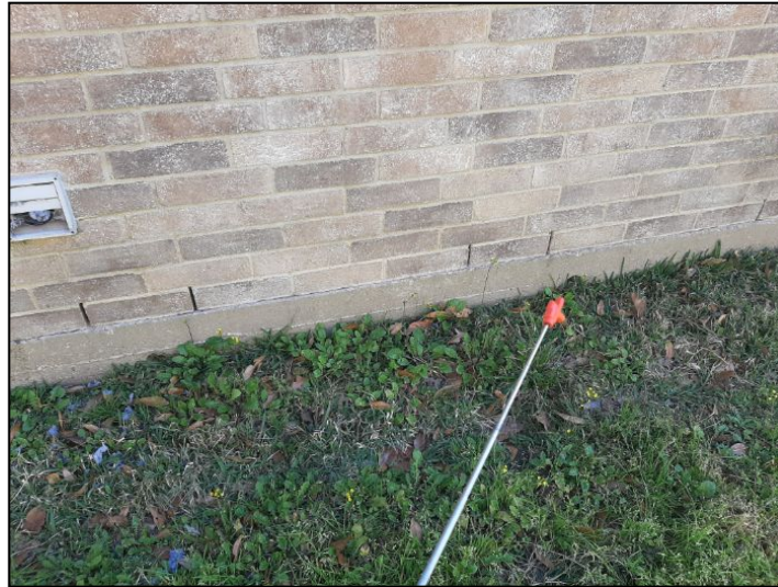
EXPOSED ANCHOR BOLTS
