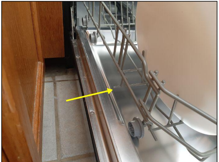
DAMAGED / MISSING ROLLER
