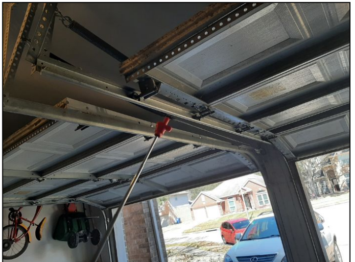
LUBRICATION NEEDED
