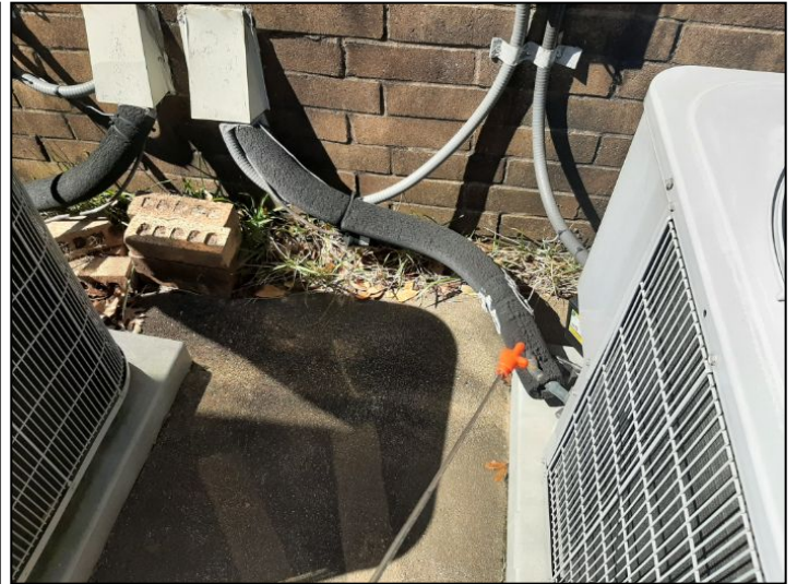
INSULATION DETERIORATION
