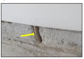
Performing its intended function. No evidence suggesting significant foundation movement at the time of inspection.
