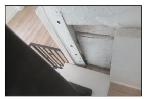
Cosmetic sheetrock damage observed in one or more areas bottom of garage wall.
