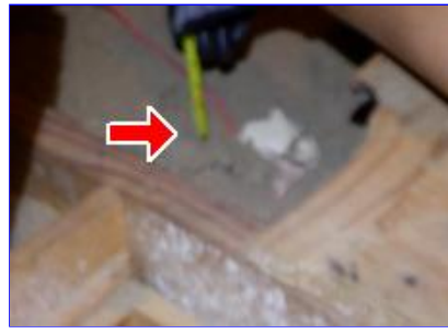
Attic insulation thickness @1"
