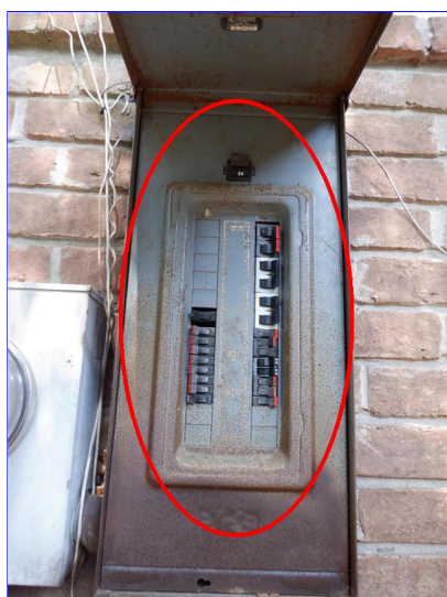
Outside main elect panel Stab Loc- FPE
