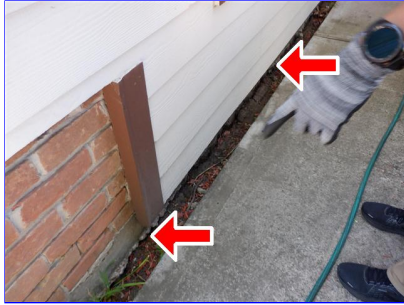
Foundation separation from soil level all around the house
