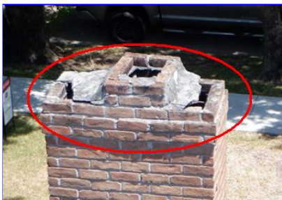
Chimney cap surface
