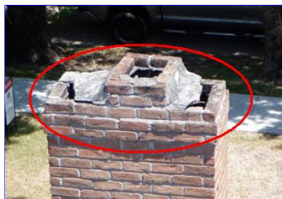
Chimney cap surface
