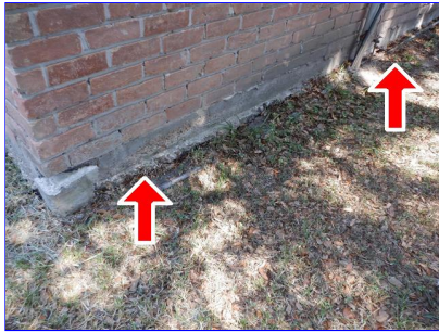
Foundation separation from soil level all around the house
