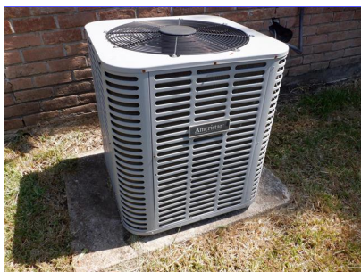
Outside AC unit,suspect 2013,9yrs old
