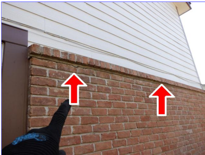
Brick wall & brick mortar separation all around the house brick walls
