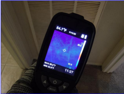
Hallway air return @84F
