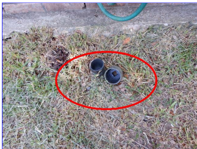
Rear main sewer drainage line
