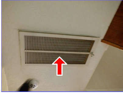
Downstair hallway air return filter replacement
