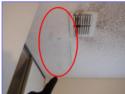
Upstair bedroom ceiling
