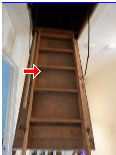
Attic stairway access
