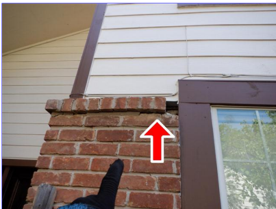
Brick wall & brick mortar separation all around the house brick walls
