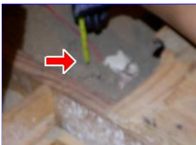
Attic insulation thickness @1"
