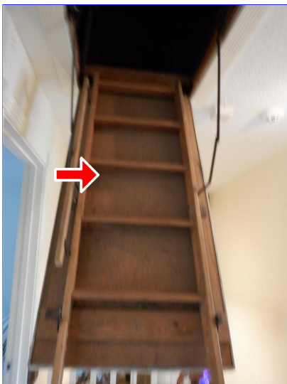
Attic stairway access
