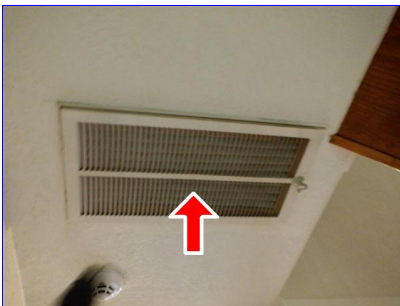
Downstair hallway air return filter replacement
