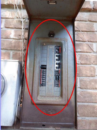
Outside main elect panel Stab Loc- FPE
