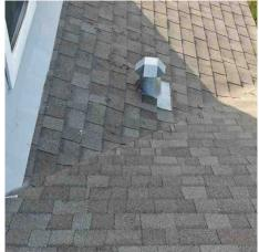
Observed un-painted portions of vent stacks through-out the roof covering. Painting of vent stacks will provide necessary UV and storm protection.
