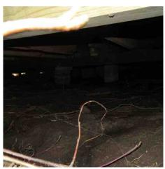
• Crawl space was inaccessible at time of inspection. No means of access could be found. Recommend installing a minimum 18" high x 24" wide access panel, as required by the International Residential **Building Code. (Throughout)**
