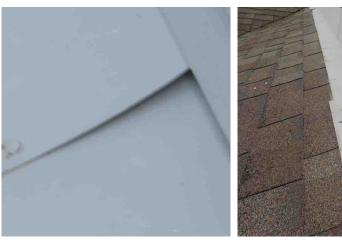
Damaged and deteriorated shingles observed at the right side roof covering (see photos below). A qualified roof contractor should examine shingles to determine if shingles are still considered serviceable. (Various)
