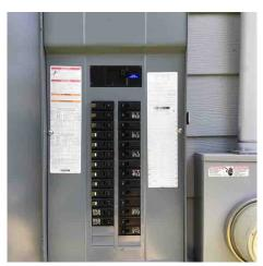
• Main distribution panel is 200 amp. Service is provided overhead from the utility company, 120/240 volt, aluminum service wires and uses breakers. Copper type wiring exist for branch circuits.
