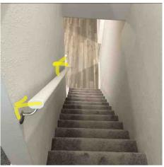
• Stair tread depth is 9". Code requires treads to be at least 10" with nosing. Recommend a qualified trim contractor construct stair in accordance with current stair safety codes. Prior to repairs home occupants should use extra care when traveling down stairs.
