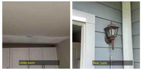
• It is recommended that this home be equipped with ground fault circuit interrupters (GFCI) at all required locations (exterior, garage, bathrooms, kitchens and within 6 feet of the outside edge of a sink). The purpose of a GFCI circuit is to provide positive protection against a shock hazard since it will "trip" almost instantaneous if it detects moisture.
