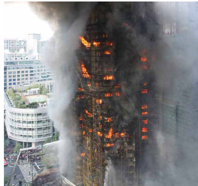
The severity of the Shanghai fire was partially a result of the use of urethane foam insulation, which aided in the spread of flame and smoke.
