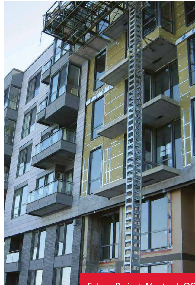
Soleno Project, Montreal, QC ROCKWOOL Cavityrock®
