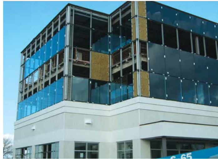
Developer Monterey Park used ROCKWOOL CURTAINROCK® insulation for its recently opened 75,000 sq. ft. commercial building in Brampton, Ontario.
