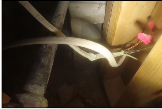
Electrical wiring in contact with gas line inside master bedroom fireplace gas starter compartment.
