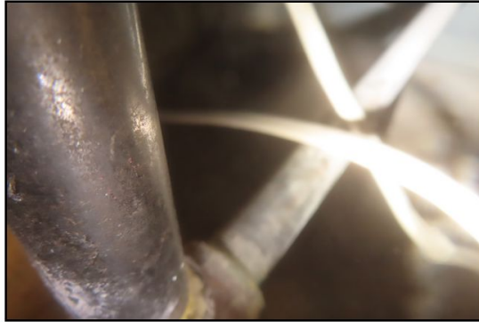
Electrical wiring in contact with gas line inside master bedroom fireplace gas starter compartment.
