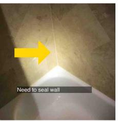
• Water leaks from the cold water handle onto the bathtub surface on the primary bathtub when the water is running, or could also be from water splashing off of the top of the tub from the faucet hitting it, needs repair.
