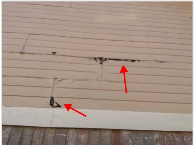
Right side exterior
