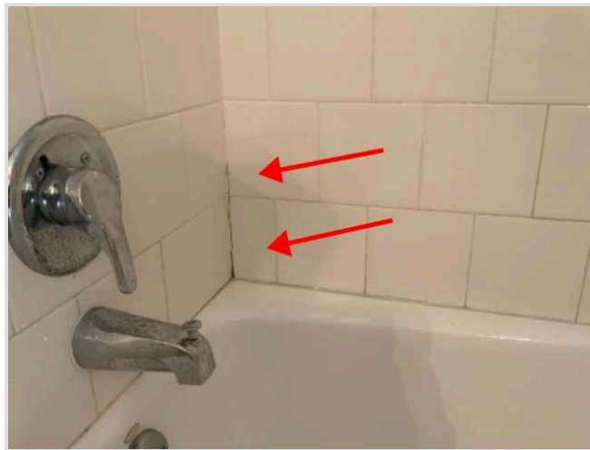
Upstairs hallway bathroom
