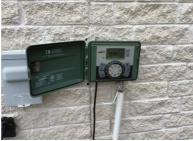
1: Valve Control not secure to wall
