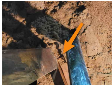
Web runners separated from the joints
