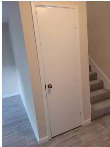
1st Floor storage door
