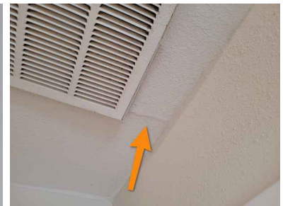
2nd Floor hallway
