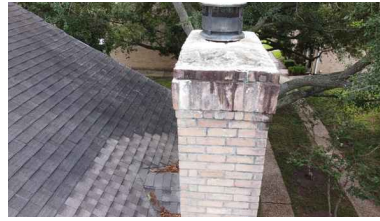
Crown, cup, spark arrestor
