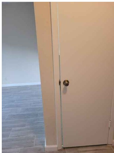
1st Floor storage door
