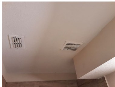
2nd Floor Bathroom
