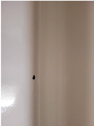
2nd Floor Bathroom
