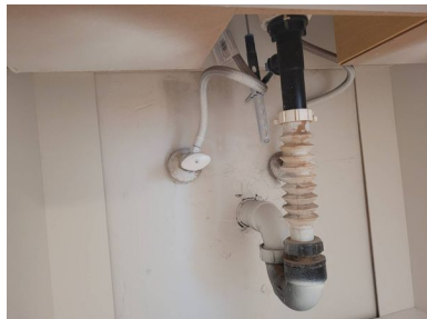
2nd Floor Bathroom
