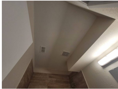
2nd Floor Bathroom
