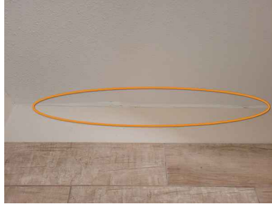
2nd Floor Bathroom
