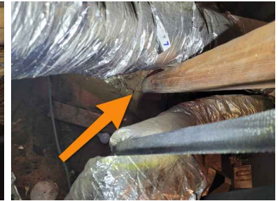
Web runners separated from the joints
