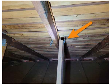
Web runners separated from the joints
