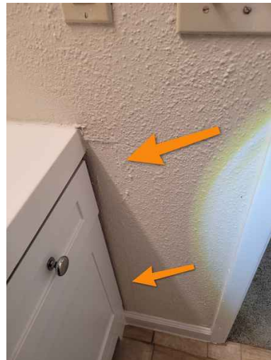
2nd Floor Bathroom
