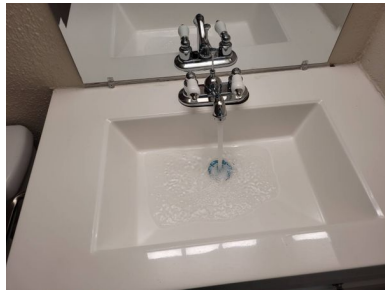
2nd Floor Bathroom
