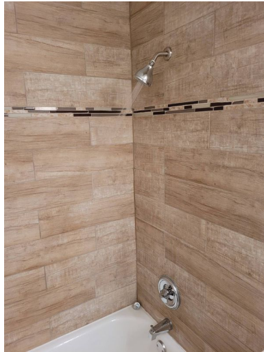
2nd Floor Bathroom
