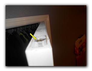
\* The doors for the master bathroom of the home hit each other when closing - need to adjust the doors to open and close properly.
