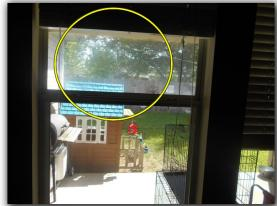
\* There is a window in the dining area of the home with a broken window pane - need to replace the broken pane for the window.
