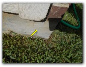
\* There is some cracking in the concrete of the garage floor of the home - this cracking is fairly common but need to monitor as this could be a sign of ground movement.
