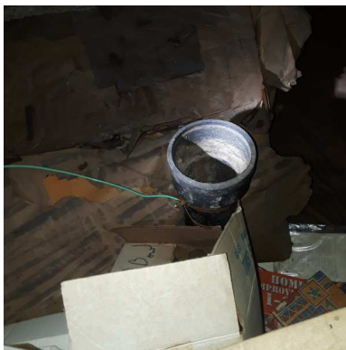
Vent into attic.
