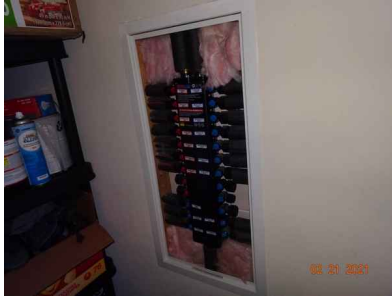
General Photo of PEX Manifold:
