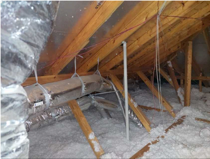
Picture of attic space
