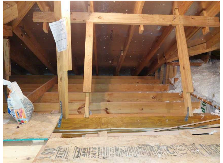
Picture of attic space
