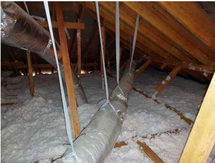
Picture of attic space
