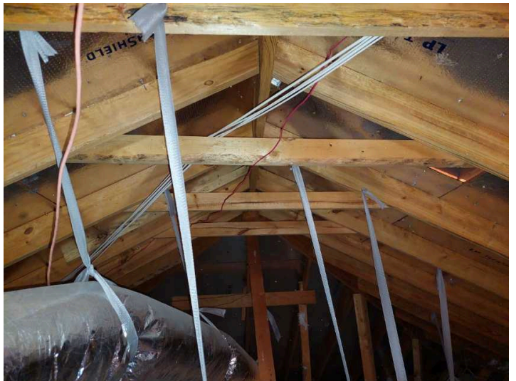
Picture of attic space
