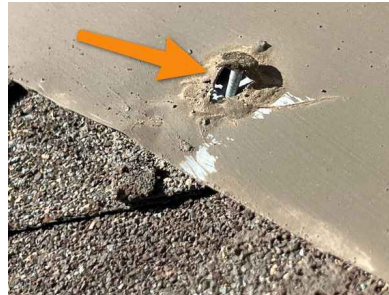
Flashing Lifting – Detail
