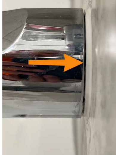
Spout Sealant Gap – Detail
