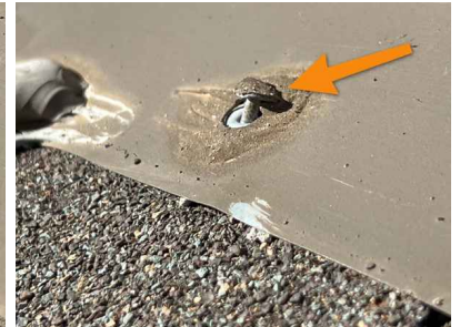
Flashing Lifting – Detail
