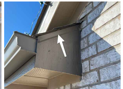
Correct Flashing (Nearby Location)
