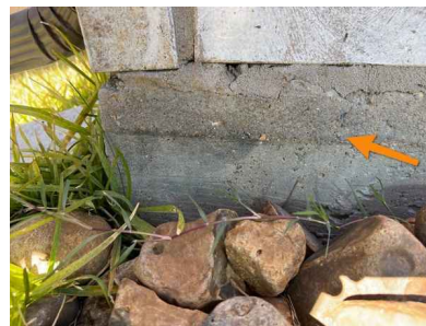
Corner Crack – Detail
