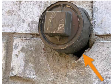
Sealant Gap – Detail
