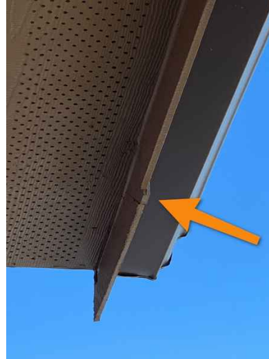
Damaged Trim – Detail
