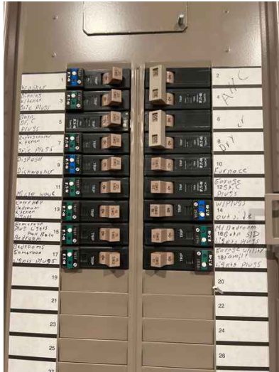
Subpanel Breakers
