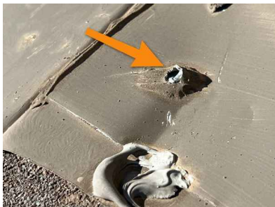
Flashing Lifting – Detail
