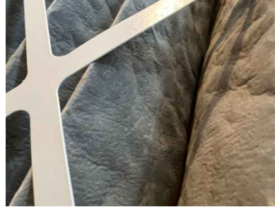
Dirty Filter – Detail
