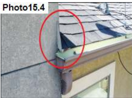
Roof Diverter Flashing / Modify
