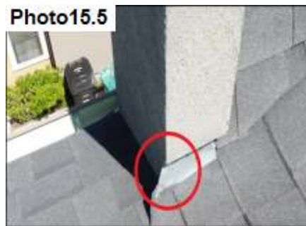
Roof Diverter Flashing / Modify
