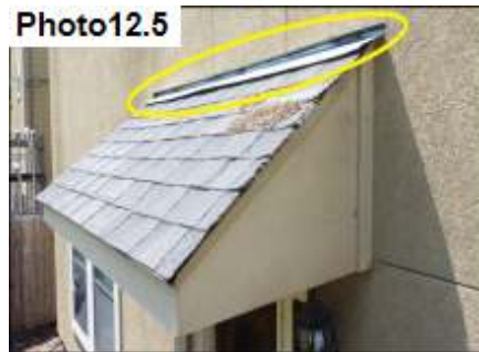
Roof Flashing / Seal
