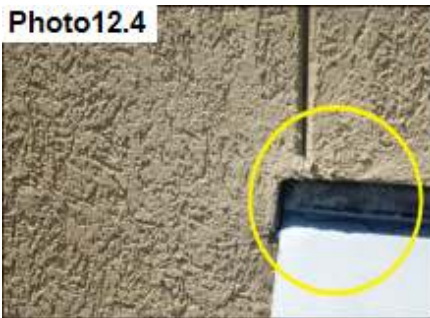
Roof Flashing / Seal
