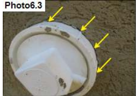
Penetration Sealants / Seal
