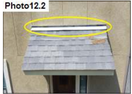
Roof Flashing / Seal
