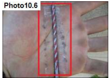
Substrate Damage / Assess & Repair
