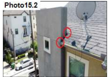
Roof Diverter Flashing / Modify
