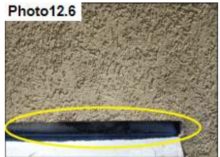
Roof Flashing / Seal
