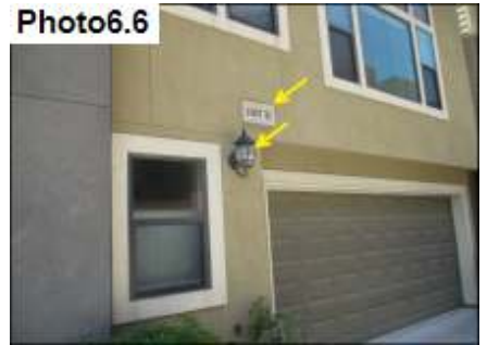
Penetration Sealants / Seal
