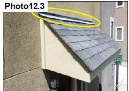
Roof Flashing / Seal
