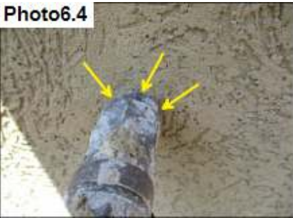
Penetration Sealants / Seal
