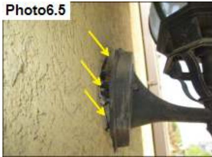
Penetration Sealants / Seal
