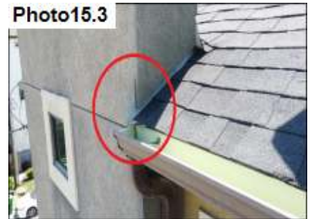
Roof Diverter Flashing / Modify
