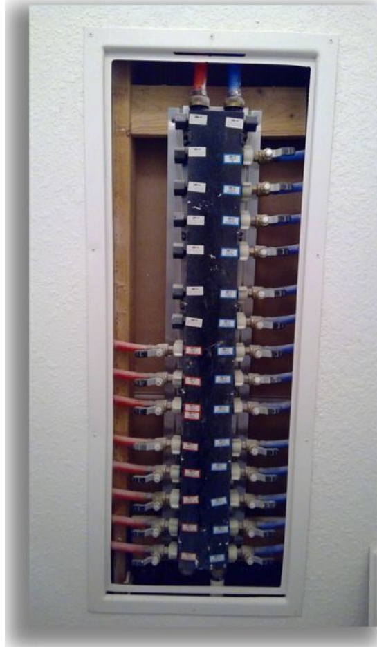
General Photo of PEX Manifold
